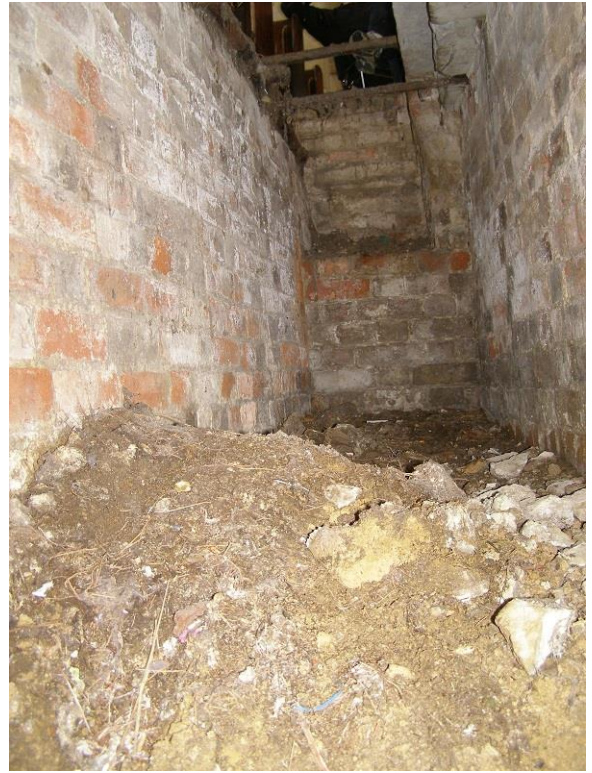
Fig 9 Entrance to north aisle duct from below
