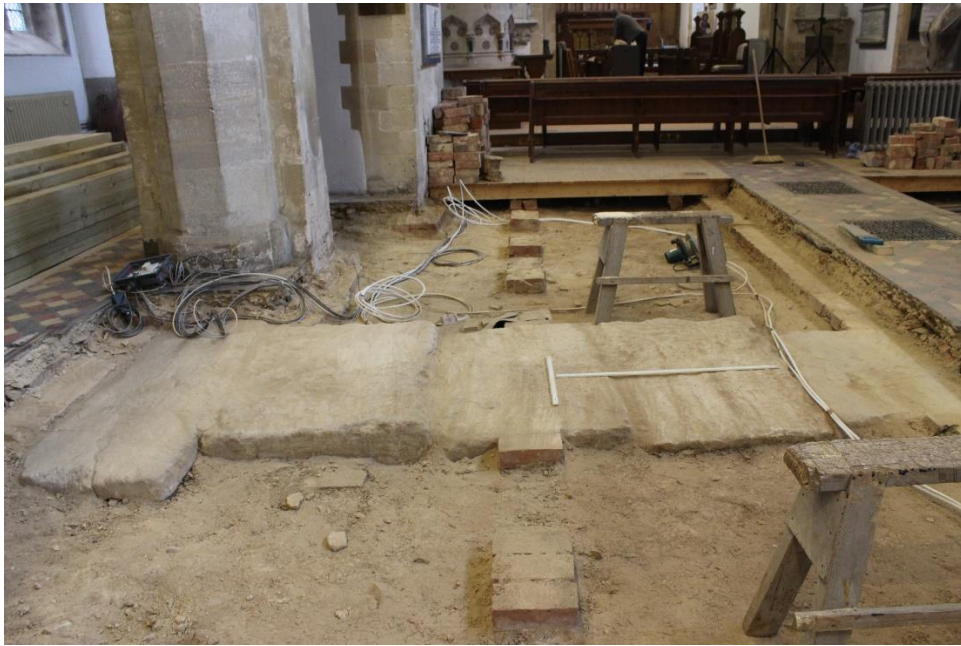
Fig 11 Massive stone slabs, possibly capping a duct across north side of nave (Scales 0.5m and 1 m)
