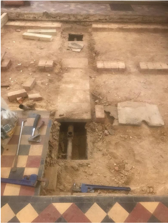
Fig 12 duct containing water pipes across south side of nave
