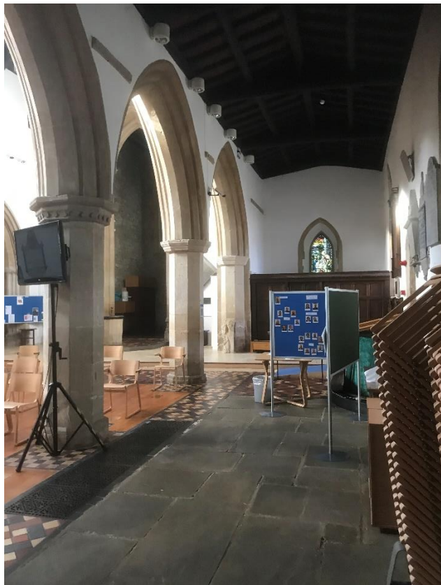
Fig 2 Nave north wall showing exterior string course pierced by aisle arcade
