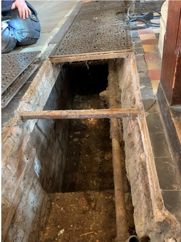
Fig 8 Entrance to north aisle duct
