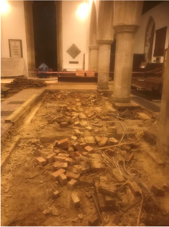
Fig 3 North pew platform removed
