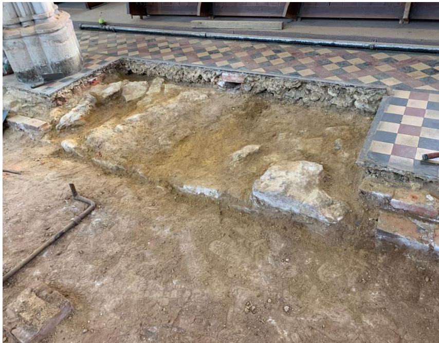
Fig. 5 South nave wall footing from north; gas pipe visible on left
