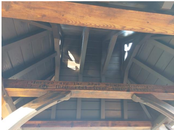
(Repaired and retained 2022)
