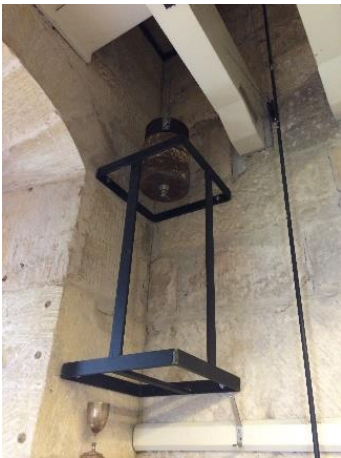
Figure 29 – Panels removed to show fabricated safety cage
