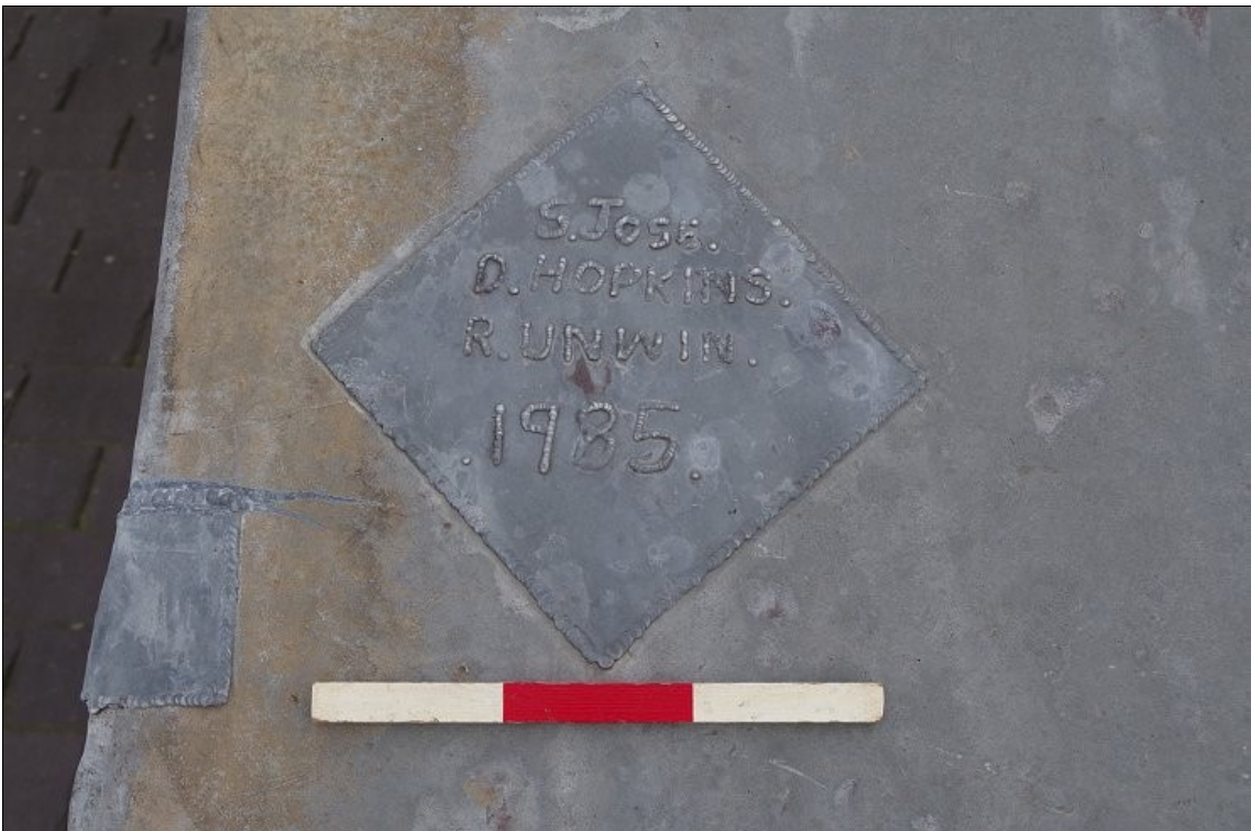
Photo 16. Lead-welded plaque commemorating roof repairs in 1985, cat. [01].
