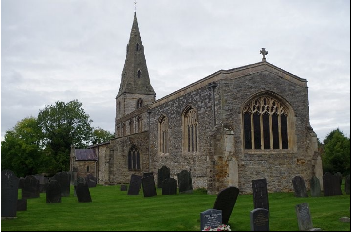
Photo 1. General view of the Church of St Mary & All Saints, looking NW.
