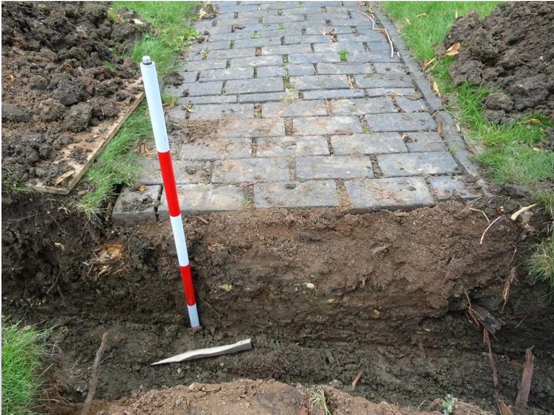
Plate 8. Trench section below a pathway, revealing eastern section
