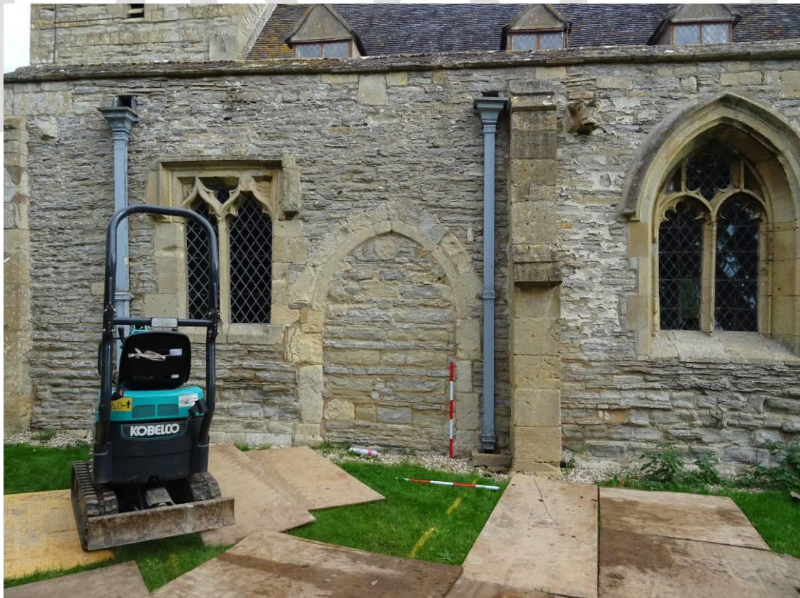
Plate 2. General view of the south aisle, looking north
