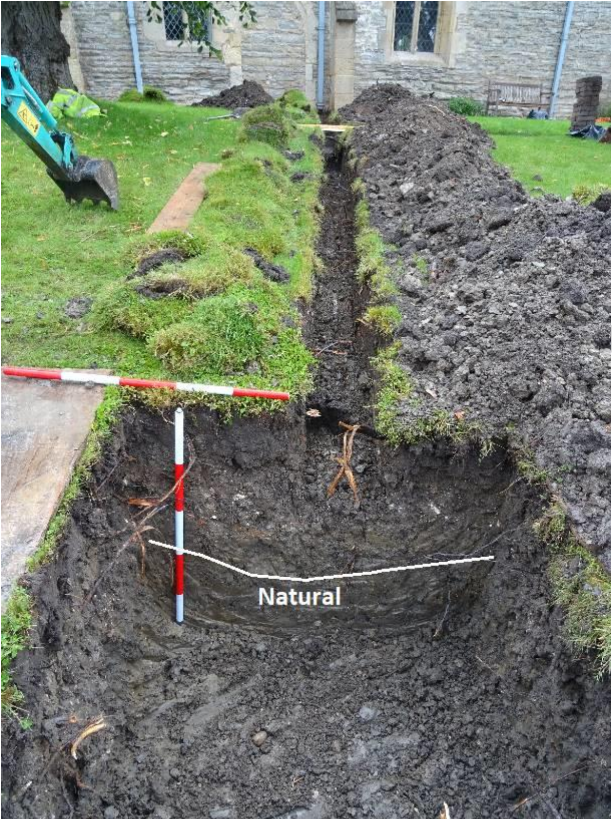
Plate 12. Full excavation of the soakaway, looking north
