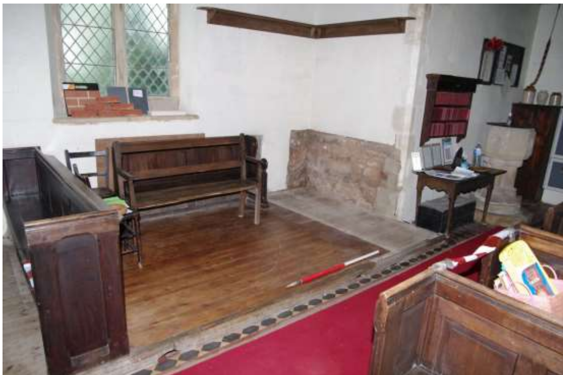
Figure 20 Pew platform in south-west corner of nave Looking south-west. 1m scale. Note font on right which will be moved
