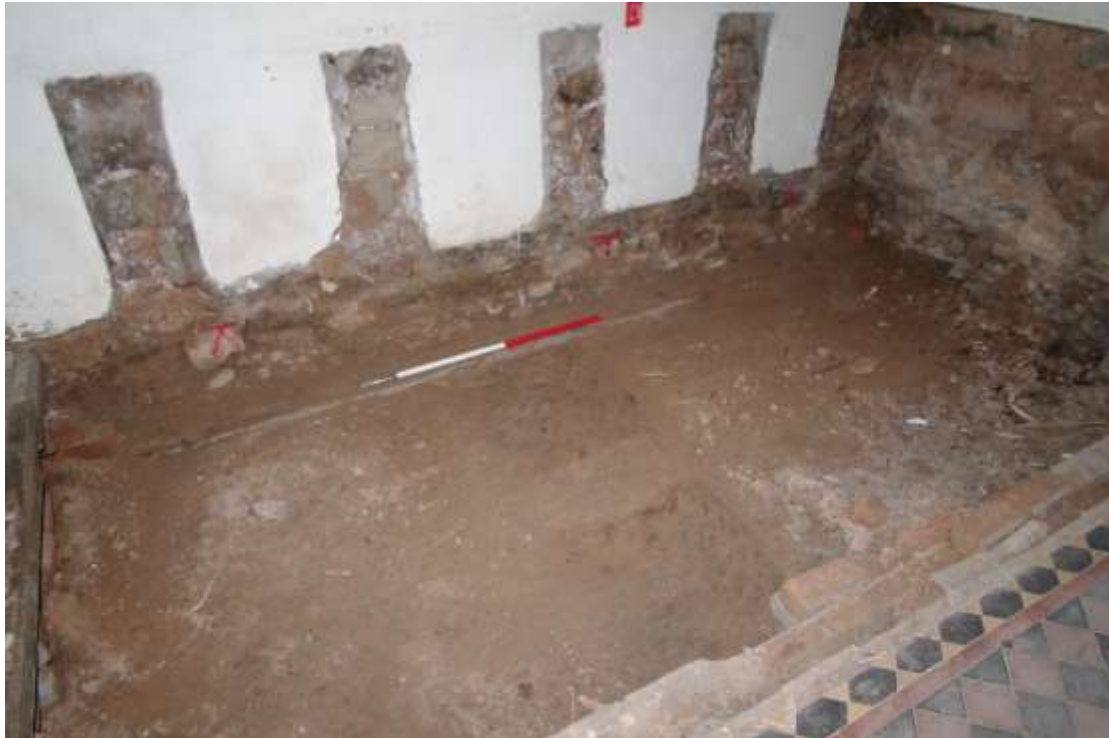
Figure 35 South-west corner of nave showing plaster outline around the pews Looking south-west. 1m scale
