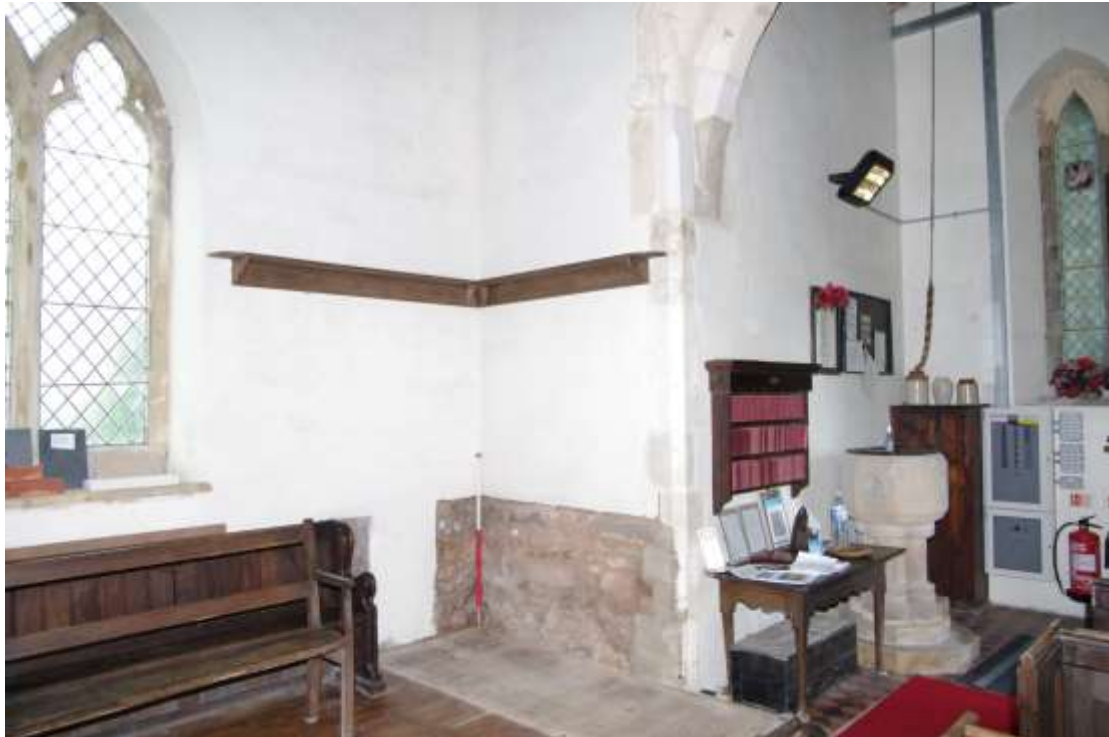
Figure 19 South-west corner of nave
