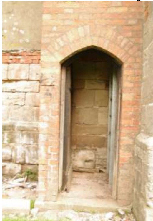
Figure 14 Open door of clock chamber and belfry access tower Looking north. The visible stonework within the doorway forms parts of a buttress which projects approximately 0.2m beyond the main wall of the tower
