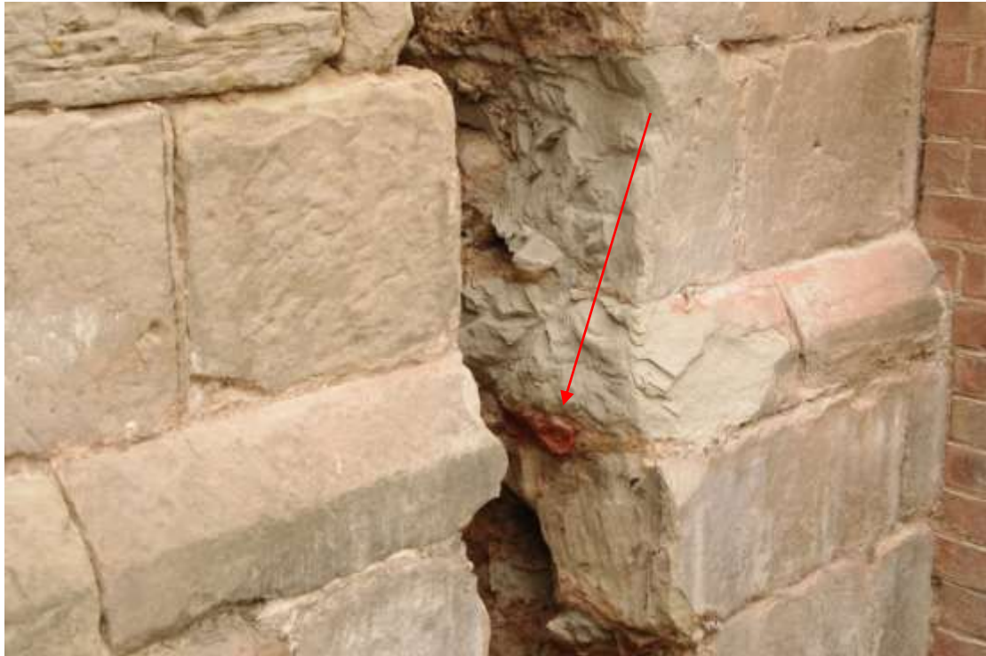
Figure 52 Fragment of brick within the stone matrix of the tower wall The red arrow points towards the brick fragment
