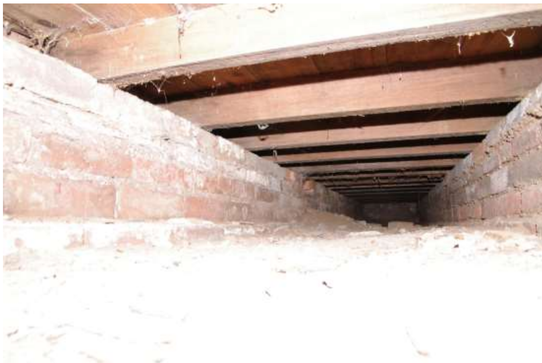
Figure 39 View beneath pew platforms Looking east
