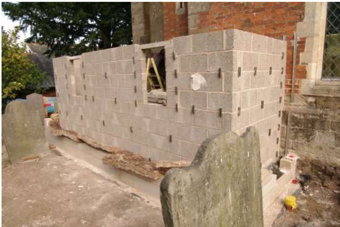
Figure 53 Partially complete extension Looking north-west
