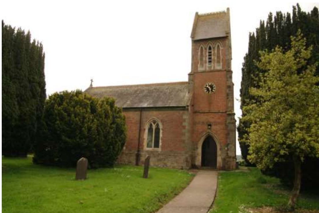
Figure 7 North facing elevation of tower A new access ramp will be added to cross the raised step into the doorway. No significant excavations will be involved for this work
