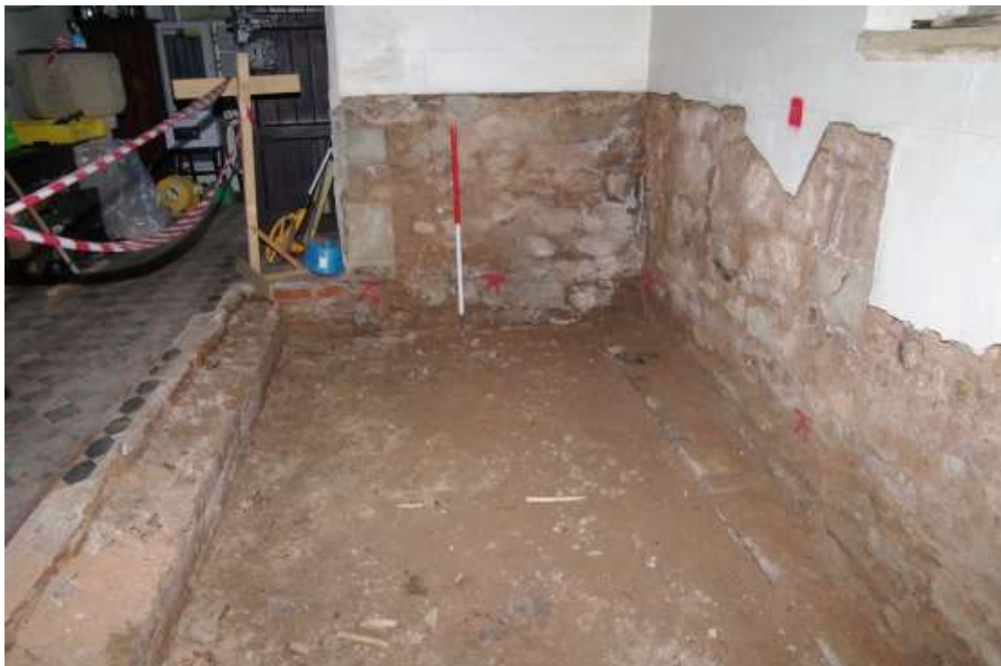
Figure 44 Tower wall on north side of aisle Looking west. 1m scale
