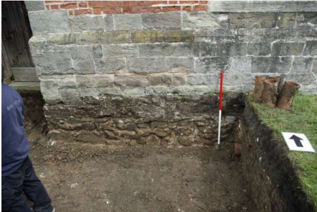
Figure 27 After removal of drain Looking north. 1m scale. The removed drainpipes are standing at the side of the trench. Note the stub of the drain extending from the side of the trench
