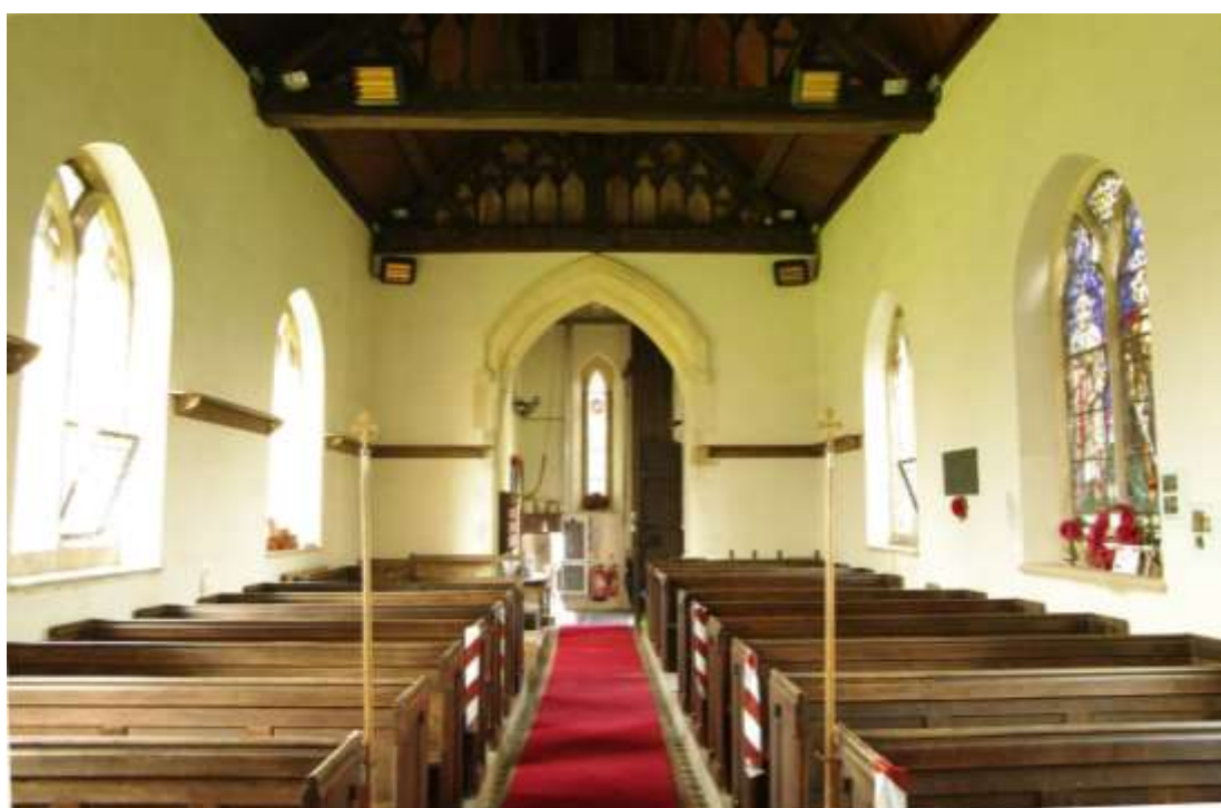
Figure 18 General looking towards the tower The furthest pews will be removed on both sides to create an open space. The font will be moved into this space
