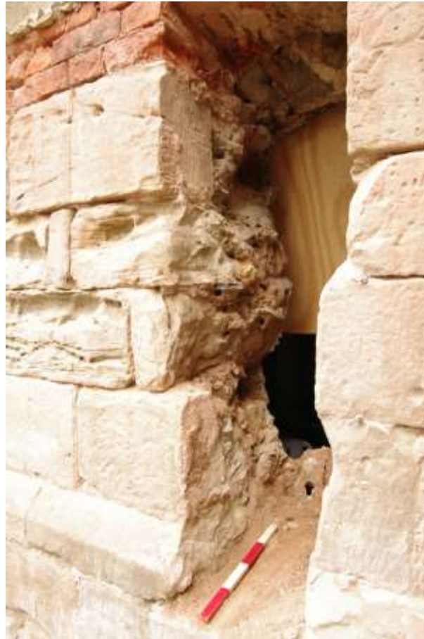
Figure 48 Slot through tower wall Looking north-west from outside. 0.4m scale
