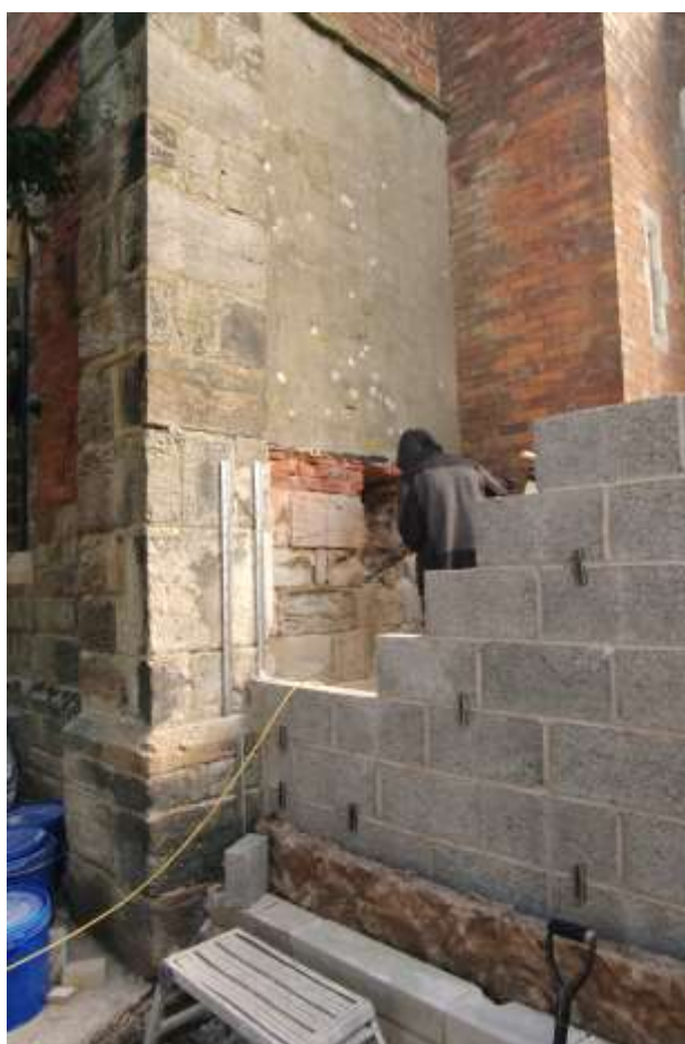
Figure 45 Initial hole being made in the south wall of the tower Looking north-east. Note the presence of the new extension by this stage
