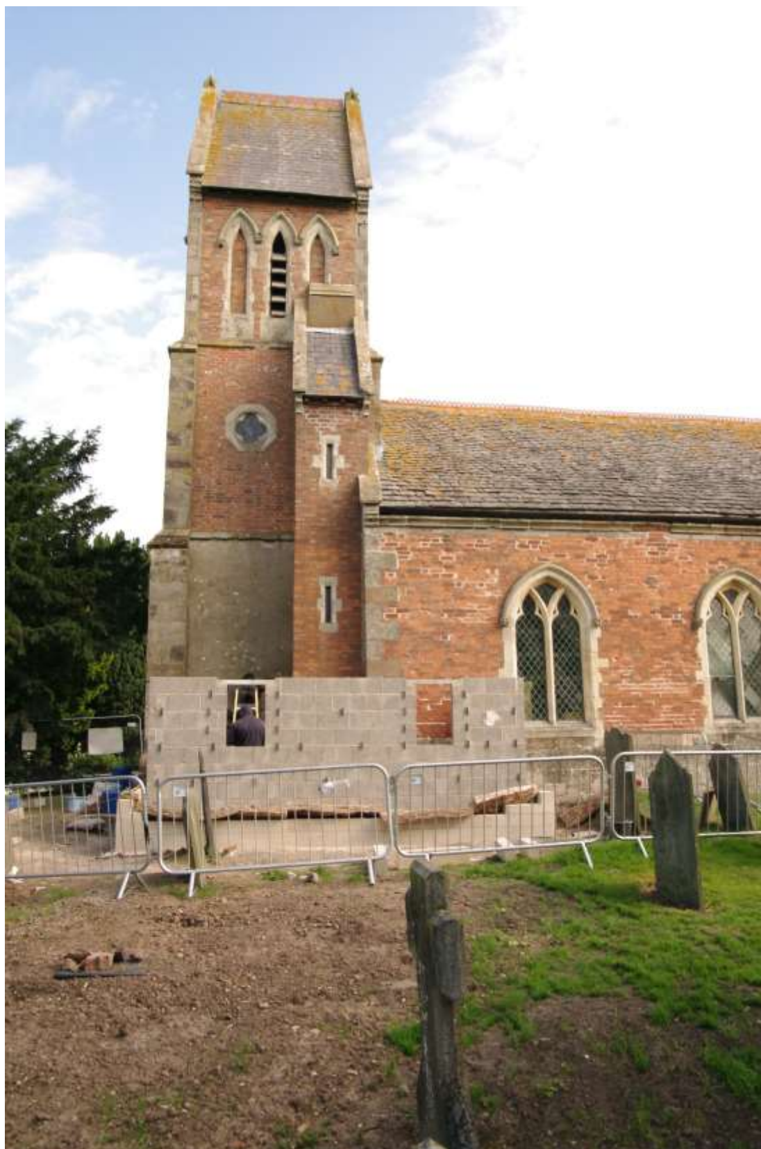
Figure 54 Partially complete extension awaiting outer skin of stone Looking north
