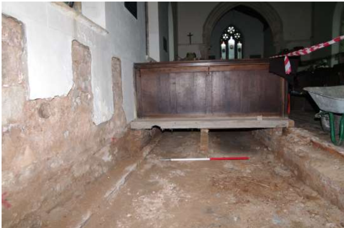
Figure 38 Supporting brickwork beneath pew platforms Looking east at pews to north of aisle. 1m scale
