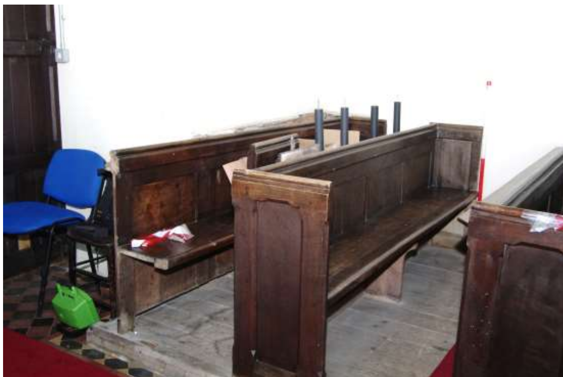
Figure 21 Pew detail on north side of nave Pews and pew platform are to be removed
