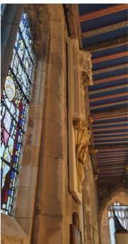
We think the monument now has a durability to its structure and that the cleaning and repair was very successful. The new stainless-steel fixings and airflow behind the plates should keep this monument in a secure and stable condition for a long time.
