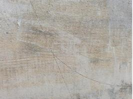
4. As the monument was mortared directly to the church wall, and the church wall appeared to be very wet for extended periods in previous years, the monument most likely absorbed a lot of the embedded salts in the wall, as clearly seen on the original scored and painted joint lines.
