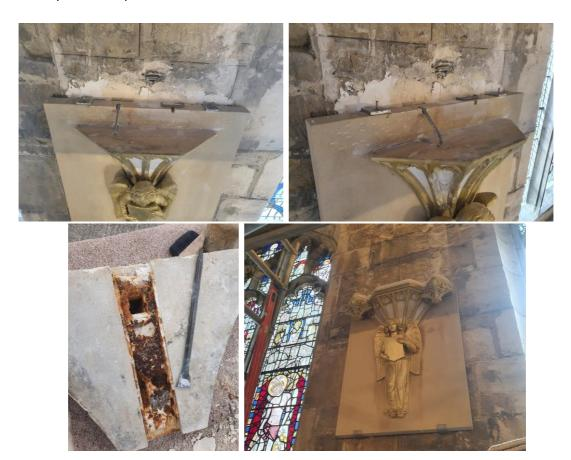
13. Above this, the shelf with two hanging corbels- which was cracked in the middle- was fitted together with two stainless steel cramps. The two hanging corbels had embedded steelwork which we removed and replaced with stainless steel. All of the carvings on this piece were heavily eroded due to salt ingress as described. All of the loose pieces were removed, cleaned and repainted with a yellow foundation paint above which was painted gold-leaf- to match the existing.
