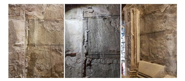
5. In short, the monument was loaded throughout with salt- which also resulted in heavy surface erosion. But some of the salt, when dried out within the cracks caused by rust jacking of the wrought-iron, grew and further accelerated the monument's decay. This indicated to us that this cracking and salt ingress has occurred over a long period of time.
