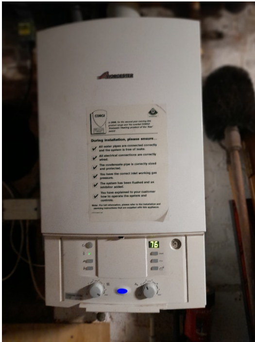
Boiler 1, Worcester Greenstar 27CDi, 27kW.
