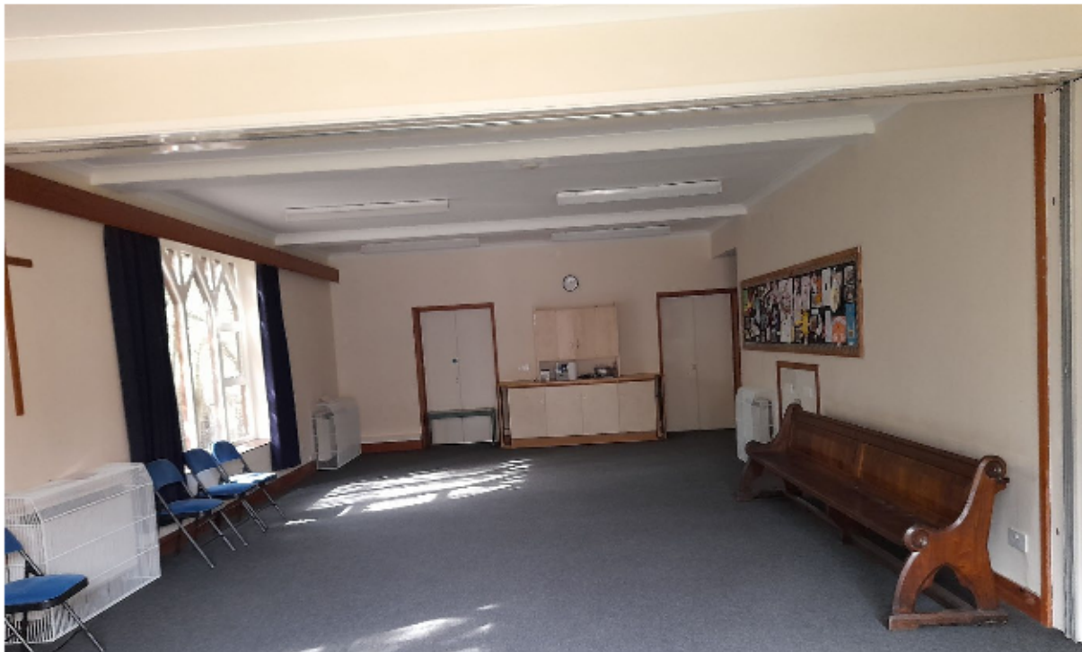
Parish Centre main room. AASHPs could be installed on the external wall to the left.
