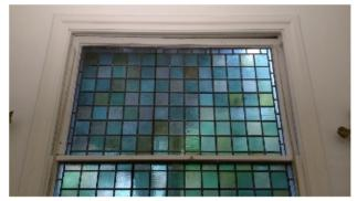
The sash window in the vestry has either dropped (see right photo at top of window) or the frame is distorted, allowing a gap and draughts. Whilst this can be sealed temporarily using plasticine, repair by a sash window maintenance company is recommended
