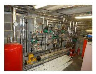
It is recommended that these a reas of expose pipework and fittings are insulated with bespoke made flexible insulation jackets. These wrap around the various elements but can be removed and then replaced for any servicing activities.
