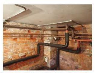
It is recommended that these areas of exposed pipework and fittings are insulated with bespoke flexible insulation jackets. These wrap around the various elements but can be removed and then replaced for any servicing activities.
