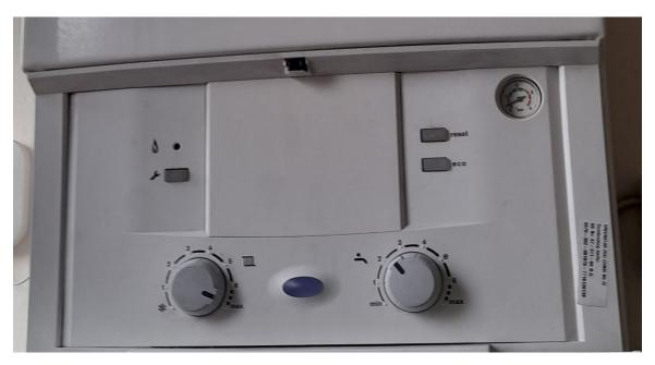
The radiators in the hall have been covered with material in an attempt to reduce surface temperature to enhance the children's safety. It is recommended that the boiler operating temperature be reduced so that the radiators are at 42°C maximum<sup>2</sup>. This will ensure that the boiler is always operating in condensing mode (below 55°C return water temperature) at
