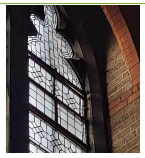
The nave west windows include four hopper openings. One opening panel is damaged; this will be allowing cold air into the church constantly, and water damage leading to deterioration of the entire window will be occurring. Repair is recommended.
