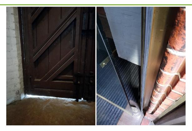
Left: The disused door at the south end of the frontage accesses the heater room – if an air intake for the heater is not provided, this gap will have to do! However, the internal door from the nave should be draught proofed.
