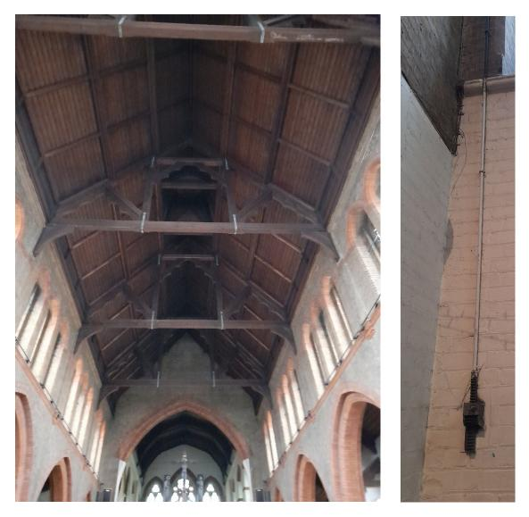
The clerestory windows in the nave have opening lights driven by a mechanism. These should be firmly closed (it is understood that they are never opened). When there is an opportunity for access and maintenance, small gaps can be filled with plasticene to ensure air tightness.
