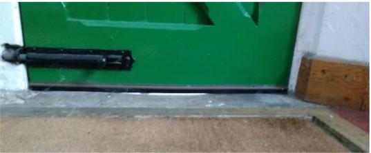
The door at the south east corner, above, is fitted with a draught strip, but it does not reach the ground where the step is worn.
