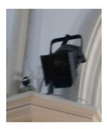
The external floodlight bulb power could not be ascertained. LED floodlights are available at 150W power. Any externally mounted lights must be IP65 rated (waterproof).
