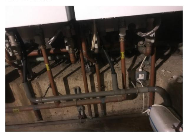
The boilers date from c. 2013, so can be expected to require repair or replacement within the next decade. In the years before the replacement of the existing heating system it is recommended that measures are taken to improve the efficiency of the existing heating system, this should include:
