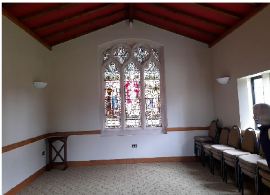
The St Mary's Room, fitted with underfloor heating.
