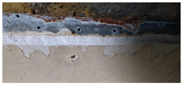
It is unclear whether this material is fibreboard, or if it contains asbestos (which it could, due to age of the boiler room building and being installed above a heat source).
