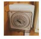
It is therefore recommended that the existing timer is adjusted to switch off the external lights between 10pm and 6am daily and also over the weekend if not required. A timeclock with a time and day capacity is recommended over those that only have time of day capacity. Sangamo (http://sangamo.co.uk/) make a wide range of commonly used timeclocks which any qualified electrician can install.
