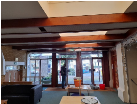
Entrance from Foley Street
