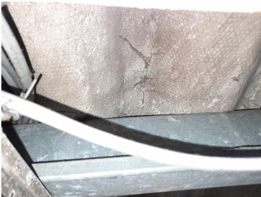
Hall roof interior viewed from first floor storage & boiler area.
