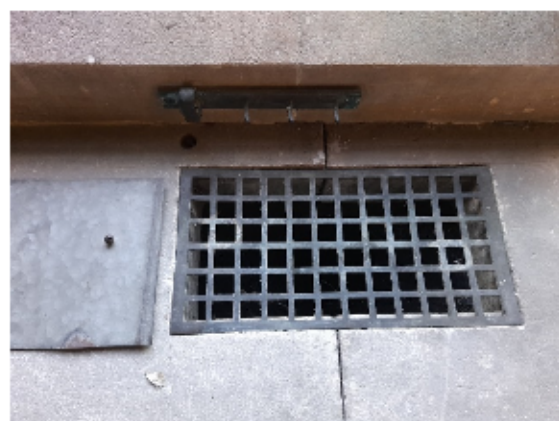
Grilles under each window allowed warm air to rise from the hidden heating pipes below.
