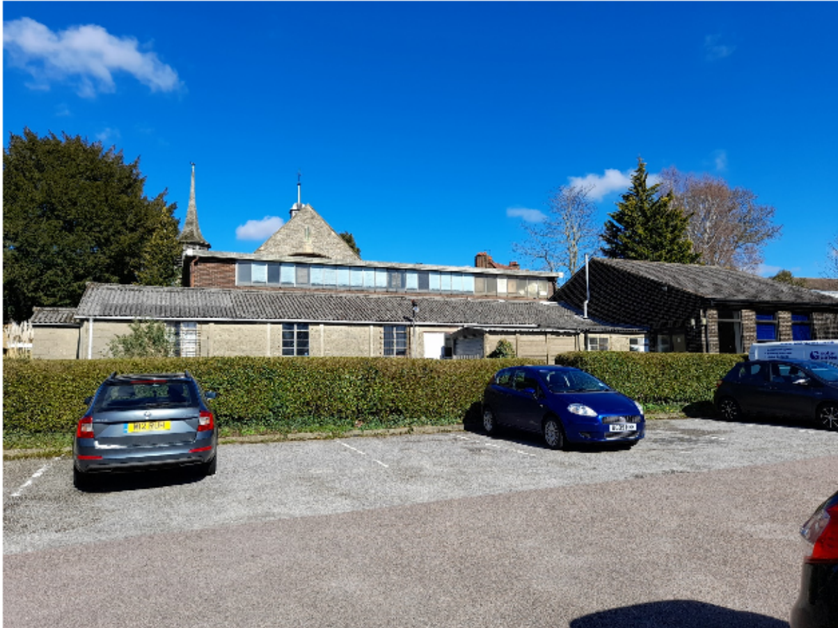
View from the south west corner of the site
