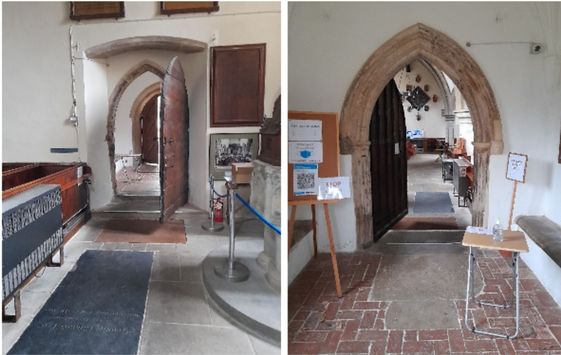
The church is entered via a porch, so good draught proofing is possible here.
