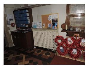
The building is heated by radiators and not all of these have thermostatic radiator valves (TRVs) installed on them, particular around the vestry area.
