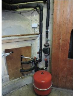
The pipework within the plant room has the majority of its straight lengths insulated but the more complex shaped pipework fittings, such as valves, have been left uninsulated. These exposed areas of pipework contribute significantly to wasted heat loss from the system and make the plant room unnecessarily warm. The exposed hot surfaces also represent a health and safety risk of burns for those working in the area.
