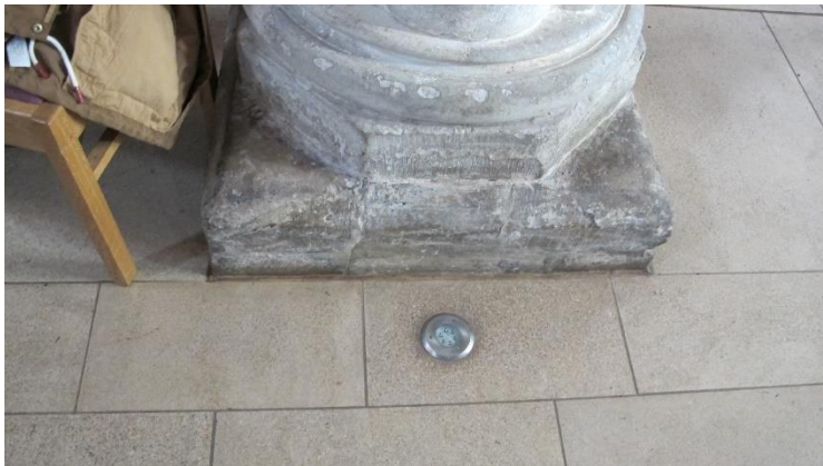
Figure 6 Recessed GU10 LED uplighter
