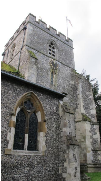
Figure 1. Showing flint construction
