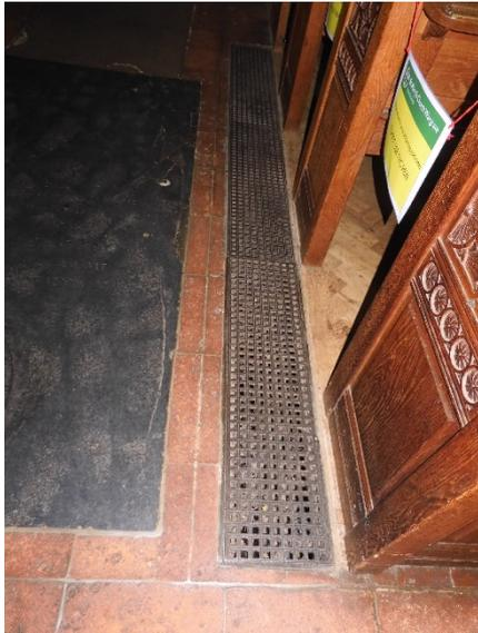
The church has a large length of metal floor grilles which used to be where the underground pipework for the heating system ran. Since the replumbing of the heating system these ducts are now redundant but they can create cold draughts which blow into the church.
