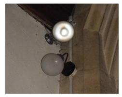
There is also a large external lighting installation which uses high energy SON lighting. As these lights are used most evenings the replacement of these to LED units is highly recommended.
