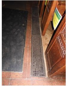
The church has a large length of metal floor grilles which used to be where the underground pipework for the heating system ran. Since the replumbing of the heating system these ducts are now redundant but they can create cold draughts which blow into the church.
