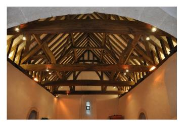
The downlights in the nave are GU10 halogen spotlights and the chancel uses PAR38 spotlights to highlight the altar. For the spot lights the Megaman range of LED spot (reflector) lights <u>https://www.megamanuk.com/products/led-lamps/reflector/</u> provides some very suitable substitutes to the current lamps.
