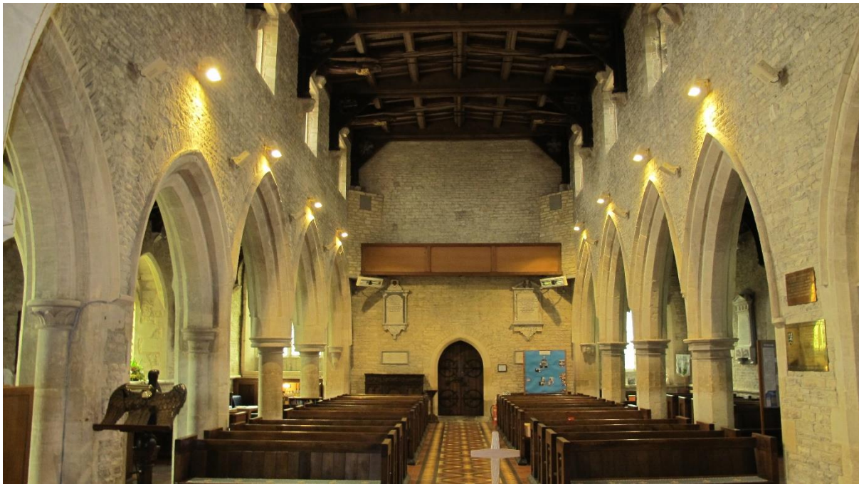
Figure 1 Nave showing lighting. Two radiant heaters on tower wall.
