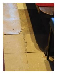
It was note that the current floor tiles are of a type which often are found to have an asbestos content and a number of these are breaking up. It is therefore strongly advised that a sample of these tiles is sent for testing without delay so that they may be managed appropriately.
