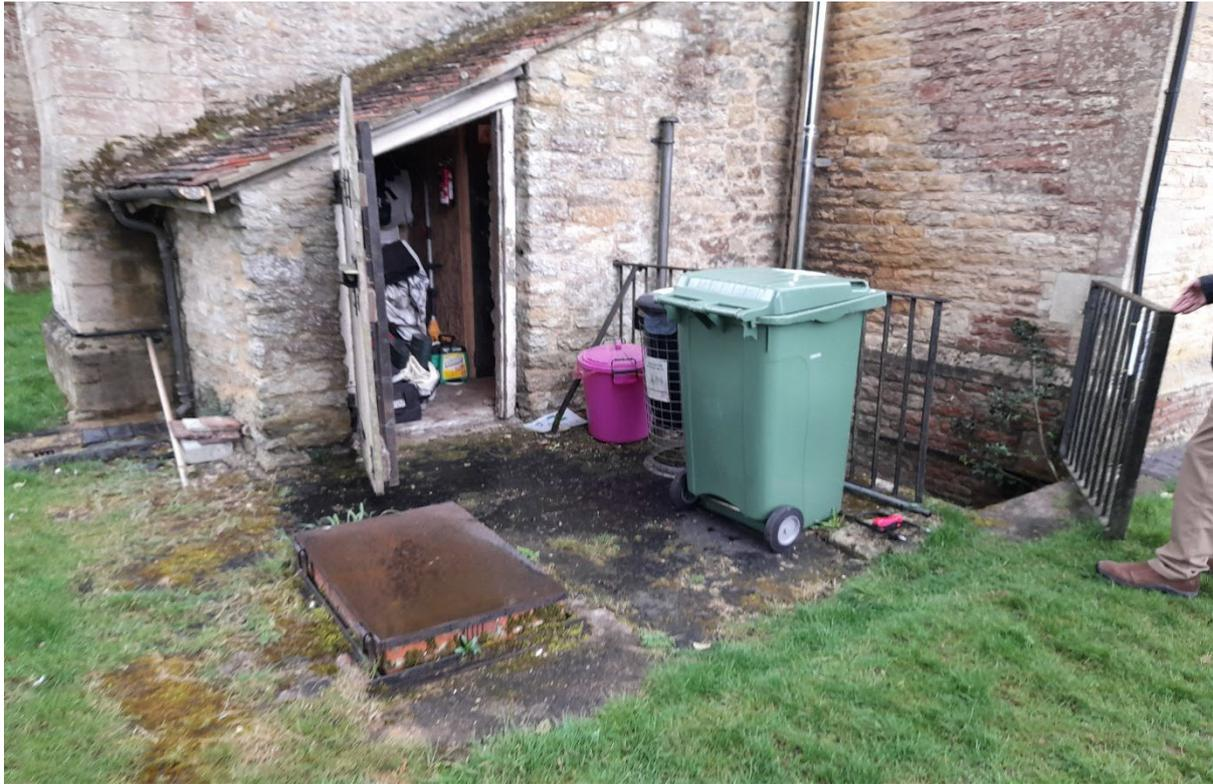
Water ingress to the coal store may be occurring through the concrete slab, or around the oil filling hatch, or the nearby drain (below).
