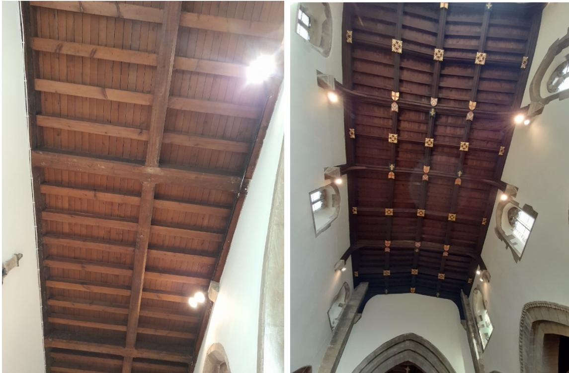
Neither aisle or nave roof are suitable for installation of rectangular panels for aesthetic reasons. The aisle beams are too close together.
