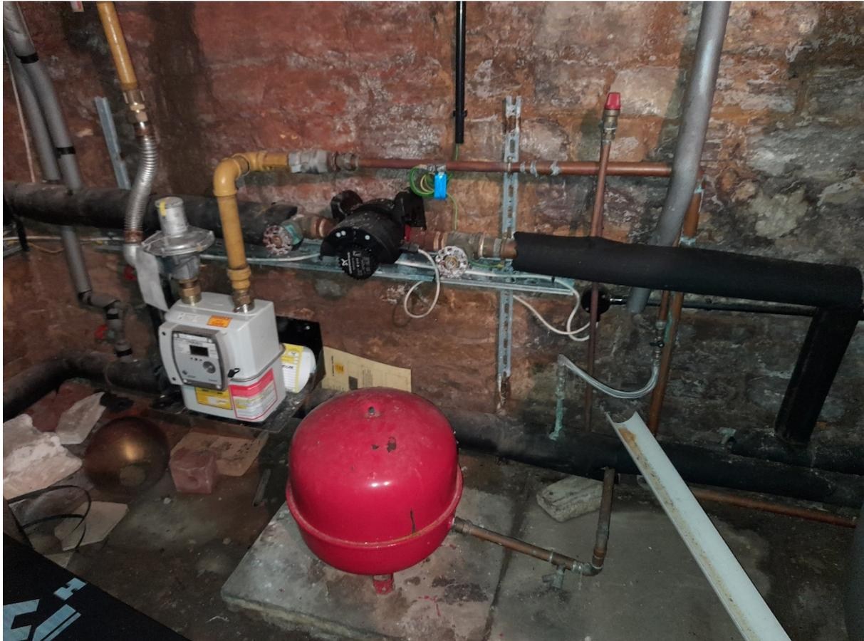
The isolation valves each side of the circulation pump have been severely corroded and cannot be turned. The red expansion tank is corroding and most of its paintwork is loose. The stopcock supplying water to the site (out of picture, above right) is corroded shut. The white guttering channels water from a leak to the drain below the condensing boiler to the right.
