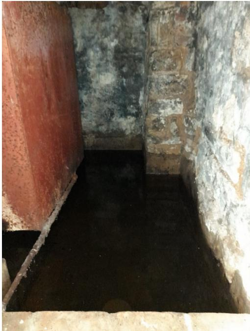
An unintentional reservoir of ground water is maintained by the low brick wall to the fore.
