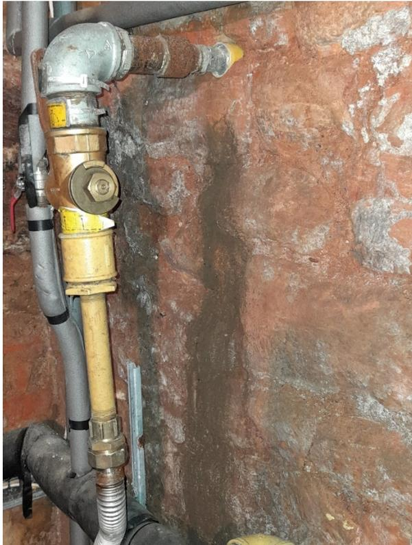
Water has been coming through the wall where the gas pipe enters. The wall was described as “crumbly”.
