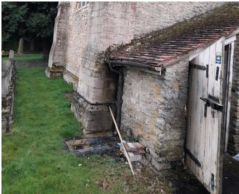
The former coal store acts as an unintentional reservoir. It is the location of the redundant, but not necessarily empty, oil tank (rusted, to the left) has collected around 40cm depth of water. This may be due to the nearby drain (above) leaking, or the gully and soakaway system which unintentionally allows a route for water to pool in this void, or it may be due to the concrete slab above the space allowing water through directly.
