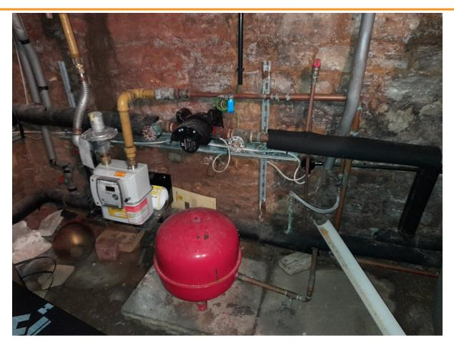
The isolation valves each side of the circulation pump have been severely corroded and cannot be turned. The red expansion tank is corroding and most of its paintwork is loose. The stopcock supplying water to the site (out of picture, above right) is corroded shut. The white guttering channels water from a leak to the drain below the condensing boiler to the right.
