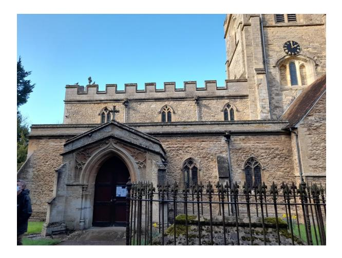
The nave and south aisle roofs are low pitched and offer sites for installation of solar photovoltaic panels which would not be visible behind the parapets.
