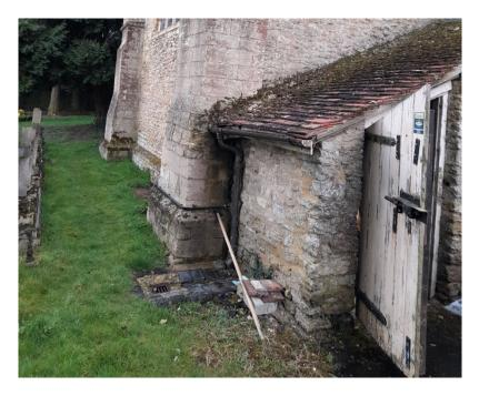
The former coal store acts as an unintentional reservoir. It is the location of the redundant, but not necessarily empty, oil tank (rusted, to the left) has collected around 40cm depth of water. This may be due to the nearby drain (above) leaking, or the gulley and soakaway system which unintentionally allows a route for water to pool in this void, or it may be due to the concrete slab above the space allowing water through directly.
