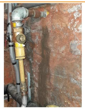
Water has been coming through the wall where the gas pipe enters. The wall was described as "crumbly".
