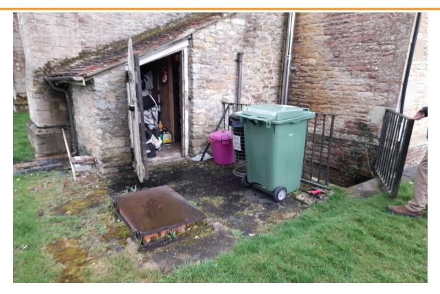
Water ingress to the coal store may be occurring through the concrete slab, or around the oil filling hatch, or the nearby drain (below).
