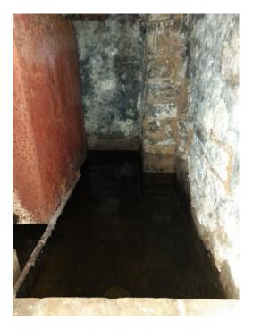
An unintentional reservoir of ground water is maintained by the low brick wall to the fore.
