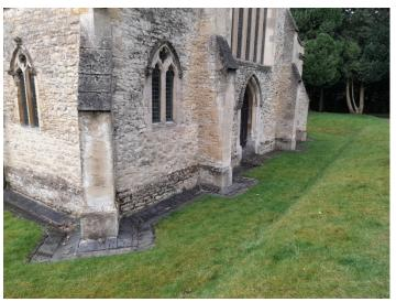
Maintaining a suitable outlet for water which collects in the stone guttering at the base of the walls (drainage ditches and soakaways) should be discussed with your Inspecting Architect.
