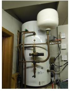
The current hot water arrangement is that there is hot water stored in a tank located in the cleaner's cupboard. This is heated up by the gas boilers in the crypt. This causes the boilers to fire twice a day every day of the year, including throughout the summer.
