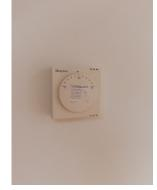
Within the church area the controls are now outdated and there are concerns that the temperature sensors are not calibrated correctly as they were reading around
