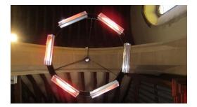
The glowing bar type radiant heaters above are clearly visible (the chandelier mounted ones can be interspersed with lighting), whereas the far infrared rectangular panels do not emit any visible radiation and can be coloured to blend in. If St Barnabas plans to retain pews, these types of heaters will be less effective than under pew heaters.
