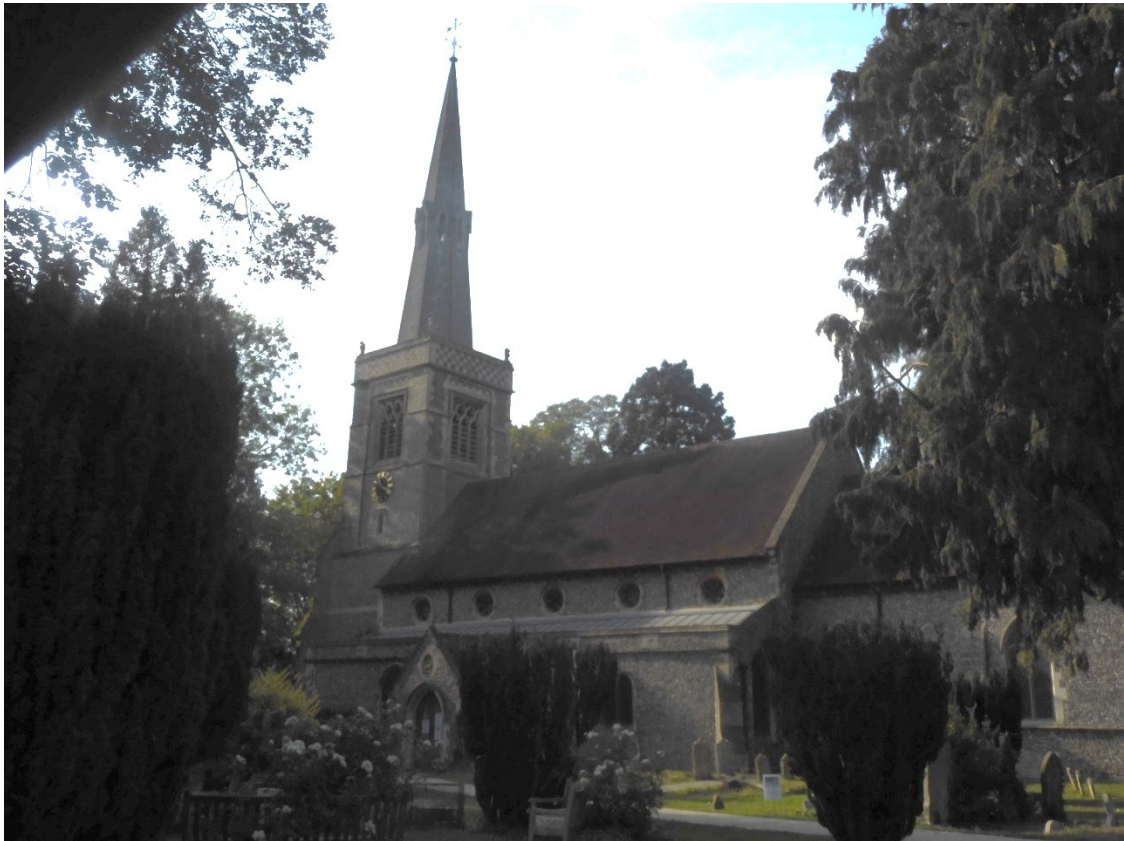
St Mary's, Princes Risborough PCC of St Mary's
