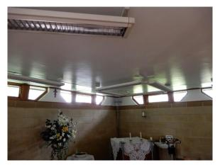
The lighting makes up a relatively small overall energy load within the building, but all areas are lit by inefficient fittings. To the main church/nave area there are three high level flood light units and to lower levels and the side rooms there are T8 fluorescent lighting and some 2D lighting.
