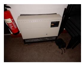
Strangely, there is the opposite issue within the two vestry areas. These small rooms have direct fired gas heaters which are flued through the wall. These have a high heat output which is too much for the space and leads to overheating in these two rooms.
