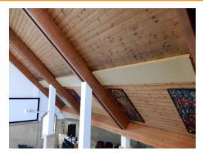
The issue appears to be that there is simply insufficient heat output from the relatively small radiant panel heaters in the main body of the church and that their positioning is such that the useful heat rises. There is then high levels of heat loss from the building, predominantly from the poor standard of windows, so that the heat input from the radiant panels is insufficient to overcome the heat loss from the building.
