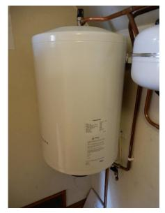
The pipework within the boiler room has not had insulated fitted to it. These exposed areas of pipework contribute significantly to wasted heat loss from the system and make the plant room unnecessarily warm. The exposed hot surfaces also represent a health and safety risk of burns for those working in the area.
