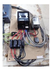
The meter is an old 2 rate dial meter and it is recommended that the church consider asking their suppliers to install smart meters so that the usage can be monitored more closely and the patterns of usage reviewed against the times the building is used.
