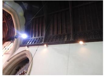
The lighting makes up a relatively small overall energy load within the building, and most areas are lit by fairly efficient fittings. The downlights in many areas are high output compact fluorescent lamps. Replacement LED lamps for these are widely available on the market and it is suggested that lamp (not the entire fitting) is replaced.
