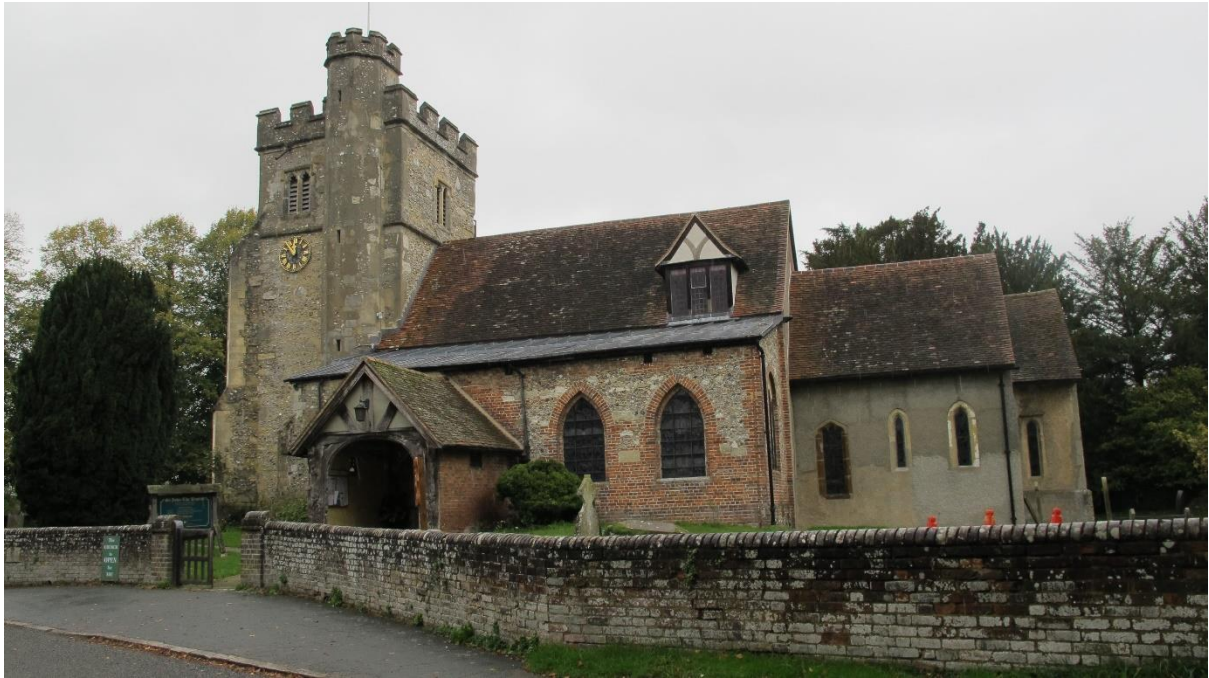
Figure 1 At 220m 2 internal area, this is a small church.
