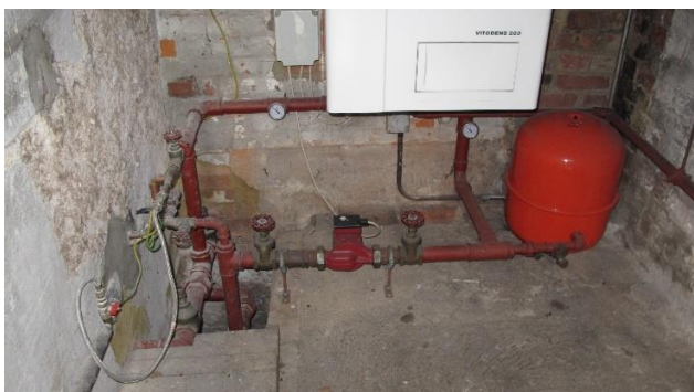
Figure 10 Unlagged pipework
