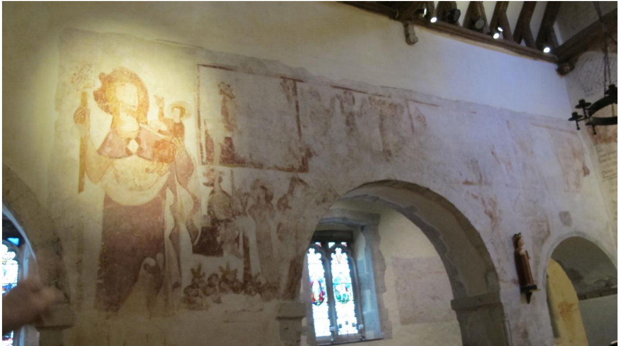
Figure 3 A recent relighting scheme has been designed to illuminate specific areas to visitors
