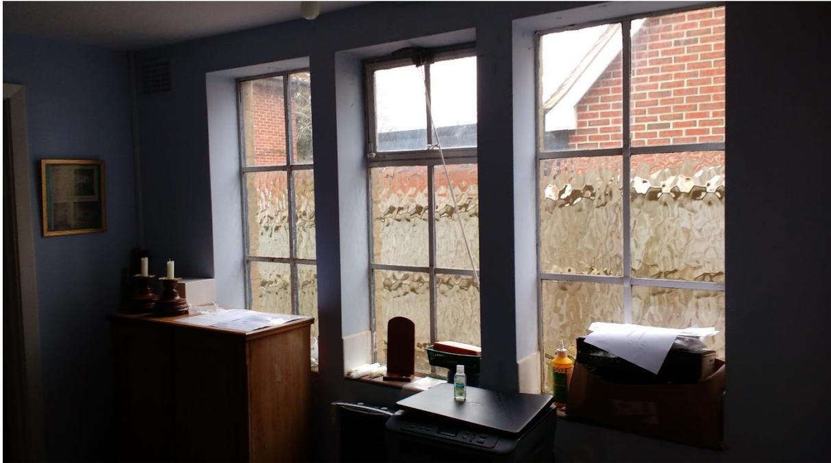
The basement area is single glazed, each area has a small portable heater. Unless it is to be used and heated regularly, there would be no benefit from installing double glazing here.
