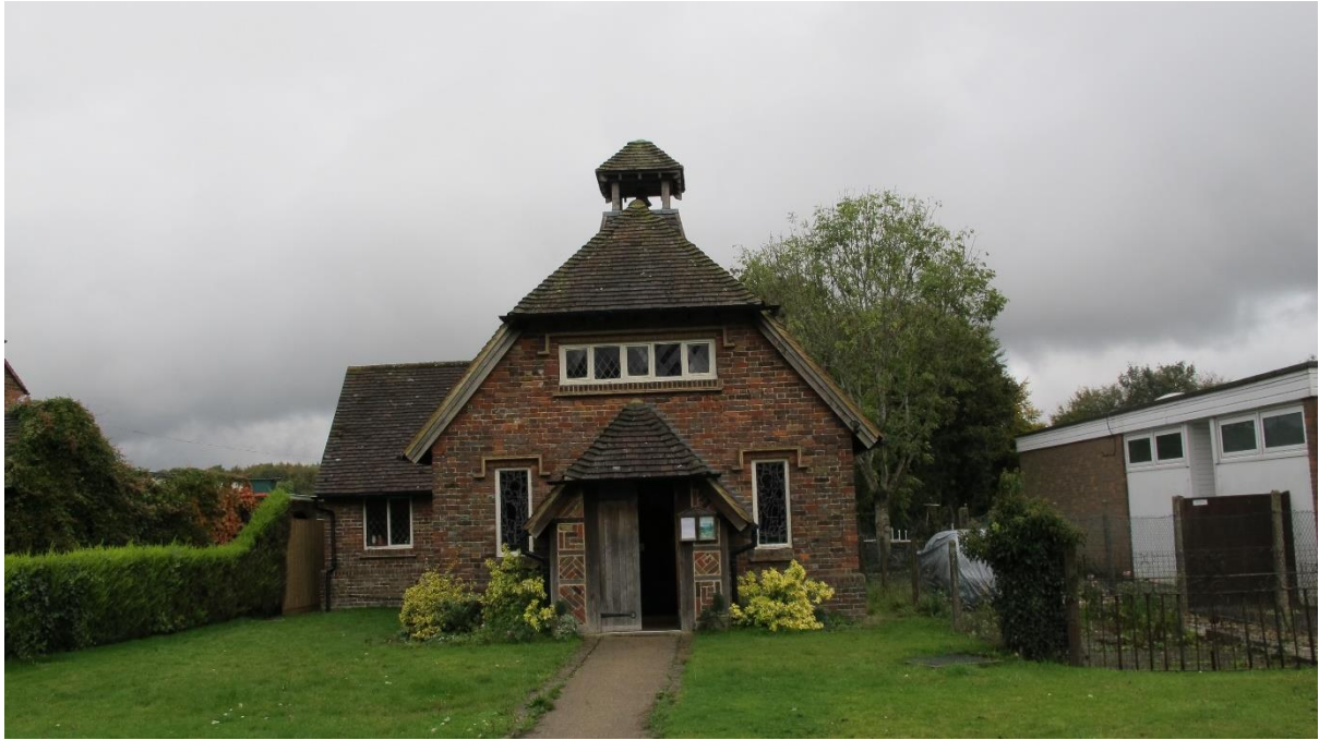
Figure 1 St Andrews's , dating from 1910, has a solid wall construction with tiled roof.
