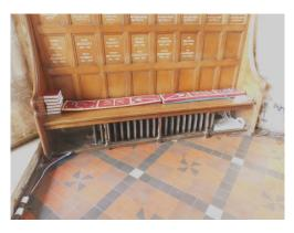
available on the market and two of these may fit under each settle which could increase the heat output and improve the distribution of heat into the nave. There is a fan noise associated with these units although at normal fan speeds this is a background hum, at boost levels it is noisier so this would be used prior to a service in a warmup period and set back during the service itself.
