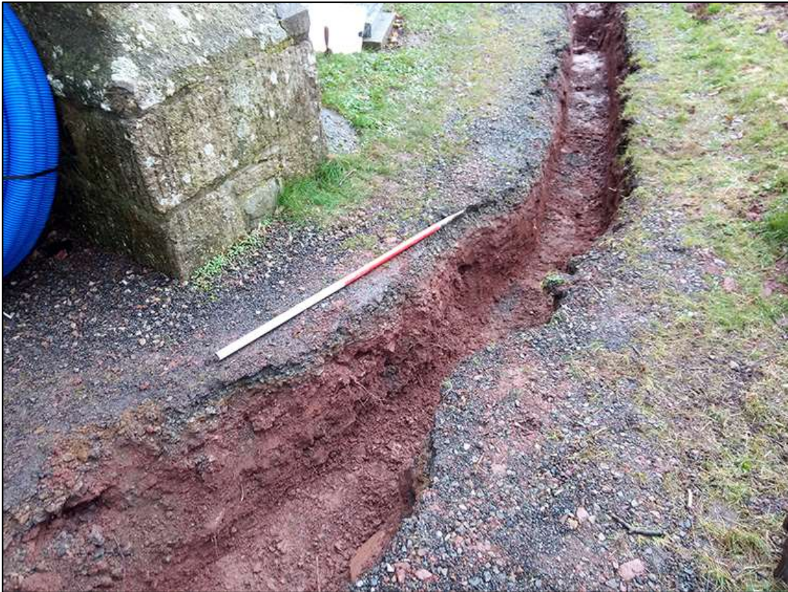
11. TOWER-SIDE SECTION OF WALL FOUNDATION {114}, POST-EXCAVATION; VIEWED FROM THE WEST (1M SCALE).
