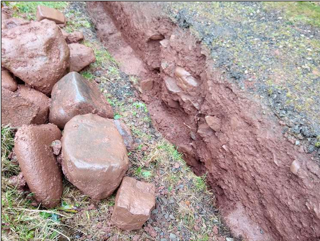
7. WALL FOUNDATION {110}, POST-EXCAVATION; VIEWED FROM THE SOUTH-EAST (NO SCALE).
