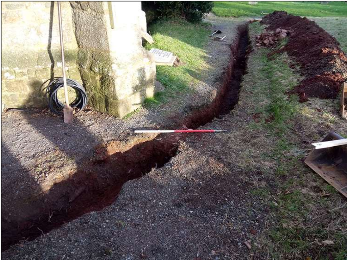
10. WALL FOUNDATION {114}, MID EXCAVATION; VIEWED FROM THE WEST (1M SCALE).
