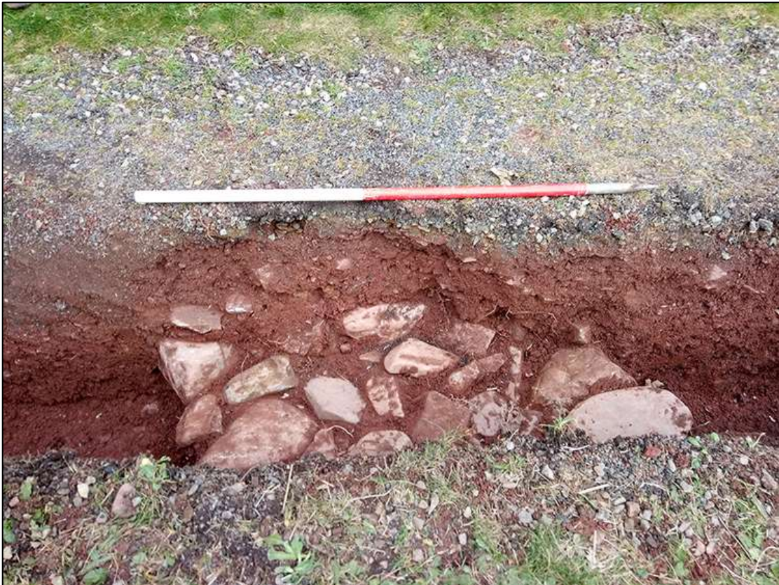
4. WALL FOUNDATION {110}, PRE-EXCAVATION; VIEWED FROM THE SOUTH (1M SCALE).
