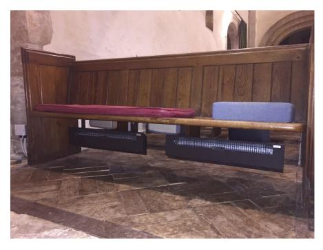
Another option is provided by "Cooltouch" fabric covered radiant under pew heaters. These are installed in St Catherine's, Towersey, a church which has additional wall mounted infra-red heaters.
