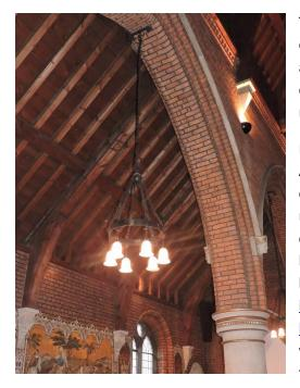
The internal lighting makes up a relatively large overall energy load within the building, and large areas are lit by relatively inefficient spot and halogen candle lights. The external lighting comprises of a number of inefficient flood lights
