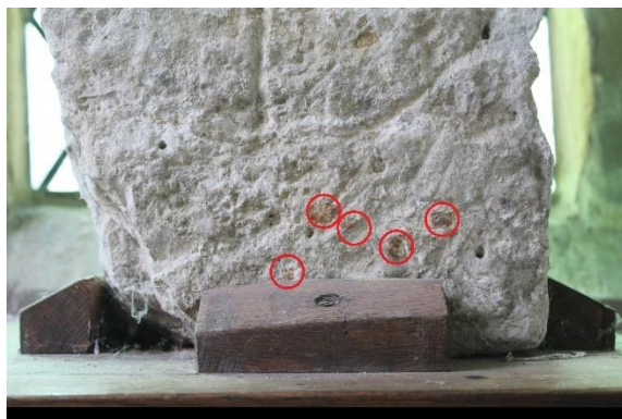
Figure 18 Location of bonded iron rust on the south face
