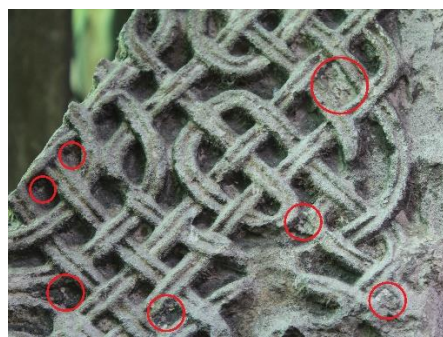
Figure 17 Location of white mortar on the west face
