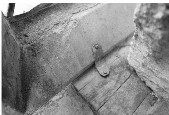
Figure 35 One of the visible attachment points from the oak box to the stone window
