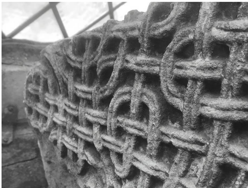
Figure 19 Carbon deposits on the west face
