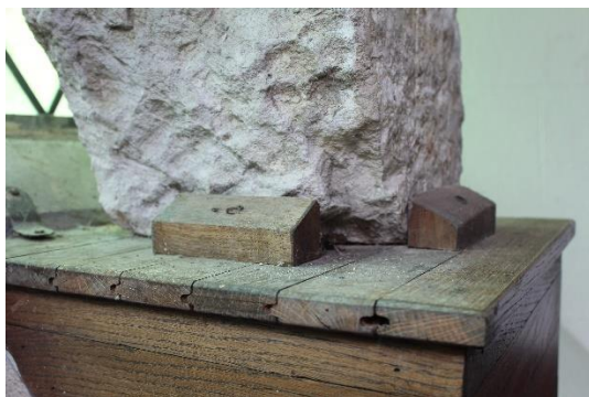
Figure 34 The wooden holding blocks around the base of the cross
