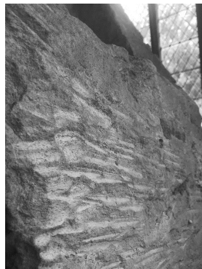
Figure 33 Cut marks made by a bolster along north side. All the decoration on this side has been lost.
