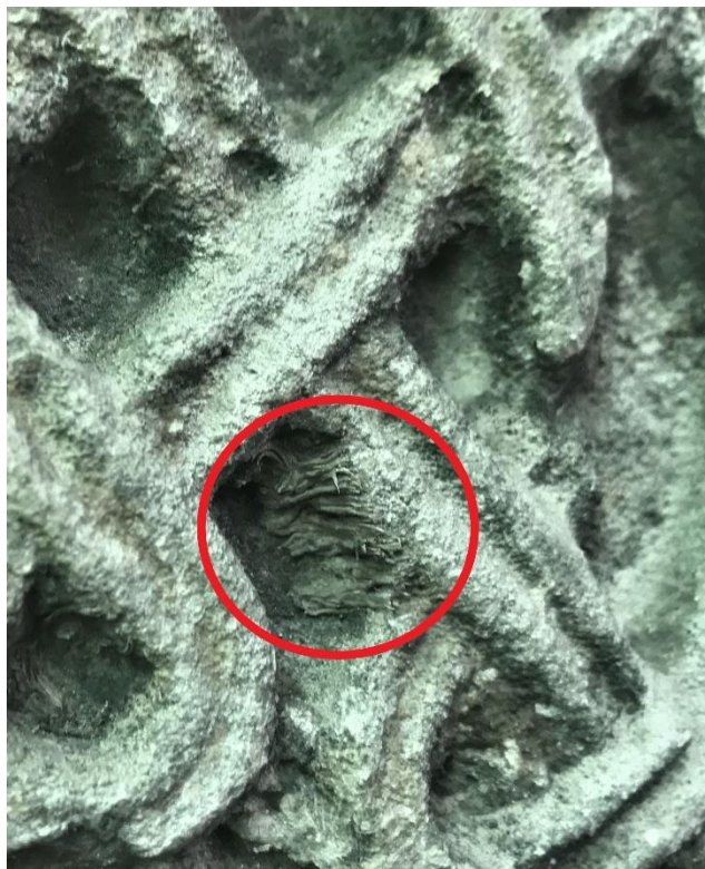
Figure 24 Detail of the root system still present from when the cross was covered with ivy
