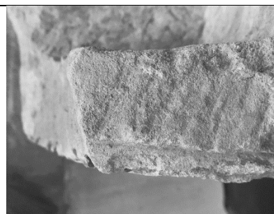
Figure 32 The top of the socket on the west side, tool marks levelling off the stone
