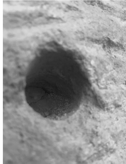
Figure 26 Detail of the northside hole, showing brown lime mortar remains within the hole
