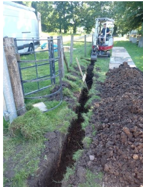
Plate 80: Excavation of the water pipe trench, from the west
