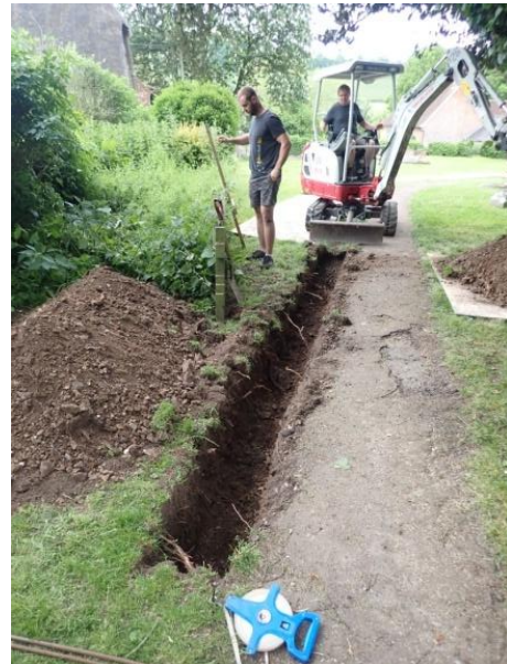
Plate 9: Excavation of the cable trench, from the north
