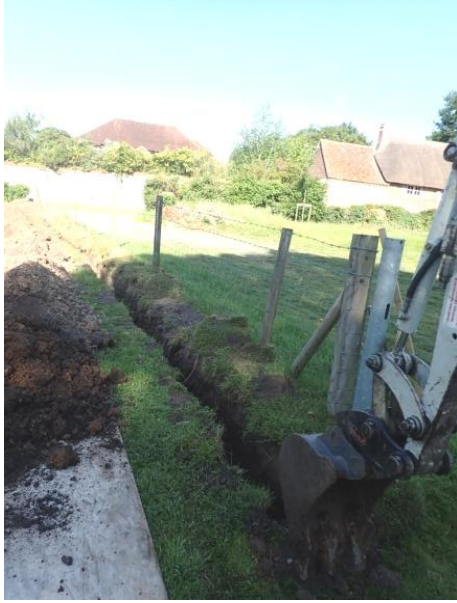
Plate 76: Excavation of the water pipe trench, from the east
