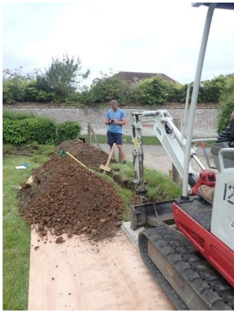
Plate 63: Excavation of the water pipe trench, from the east
