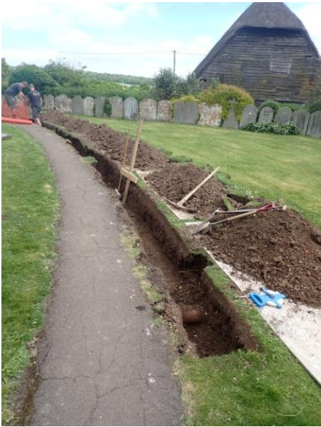
Plate 17: Excavation of the cable trench, from the west
