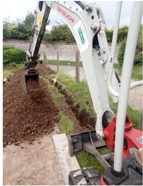
Plate 64: Excavation of the water pipe trench, from the east
