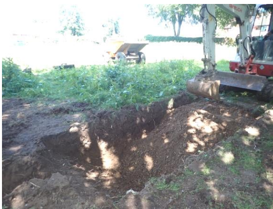
Plate 110: Excavations for the septic tank, from the east
