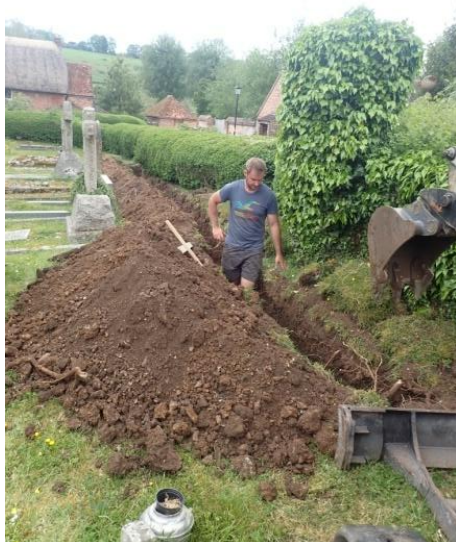
Plate 57: Excavation of the water pipe trench, from the north
