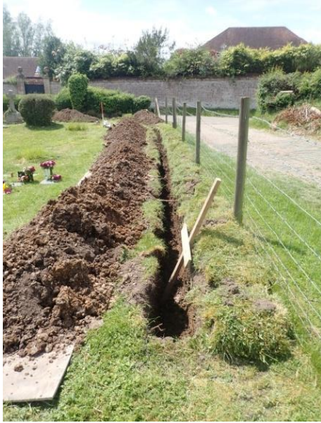
Plate 71: Excavation of the water pipe trench, from the east
