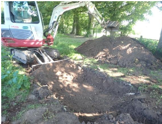
Plate 103: Excavations for the septic tank, from the south-west
