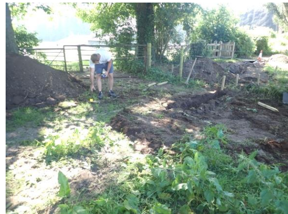
Plate 101: Excavations for the septic tank, from the west
