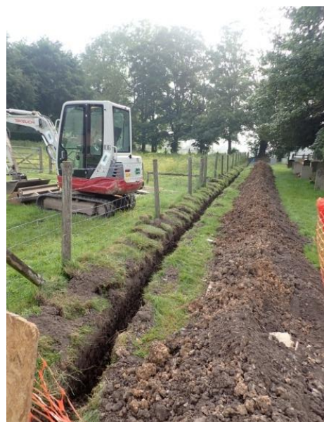
Plate 95: Excavation of the water pipe trench, from the west
