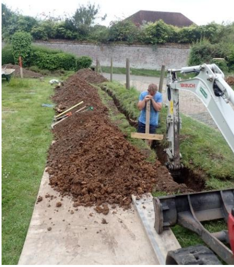
Plate 66: Excavation of the water pipe trench, from the east
