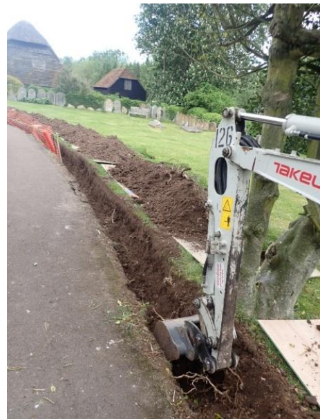
Plate 23: Excavation of the cable trench, from the west
