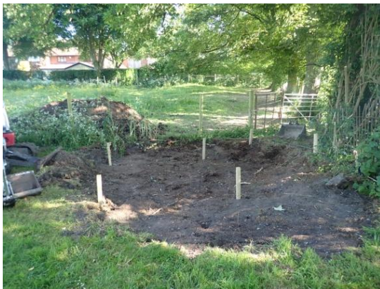
Plate 48: Excavated toilet block site, from the south
