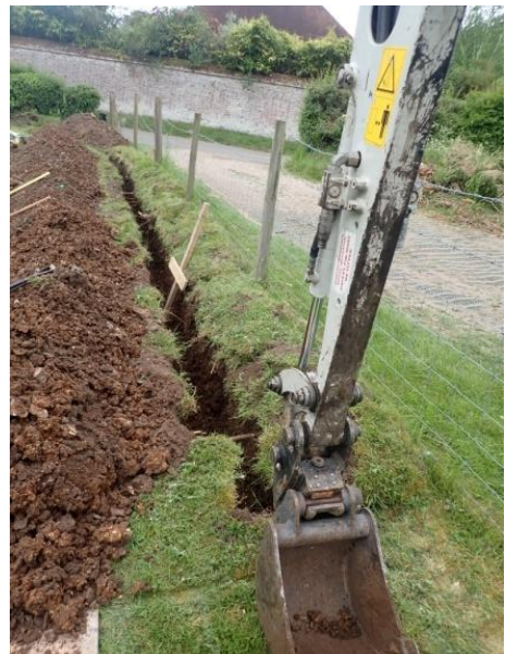
Plate 70: Excavation of the water pipe trench, from the east
