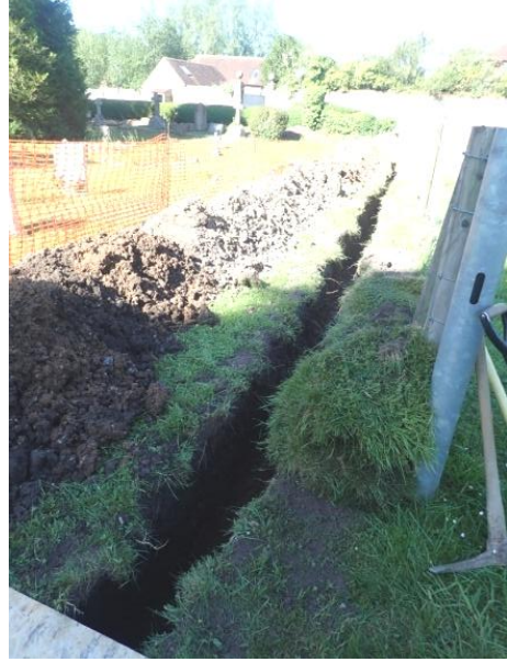
Plate 78: Excavation of the water pipe trench, from the east
