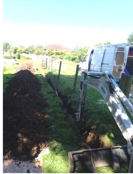
Plate 83: Excavation of the water pipe trench, from the east
