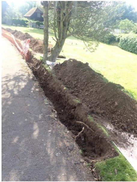
Plate 24: Excavation of the cable trench, from the west
