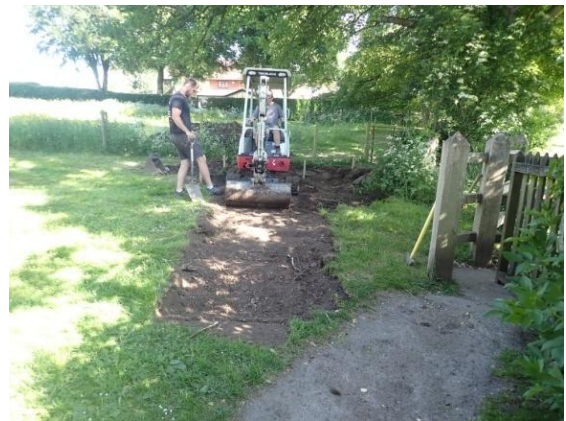
Plate 45: Excavation of the cable trench, from the south
