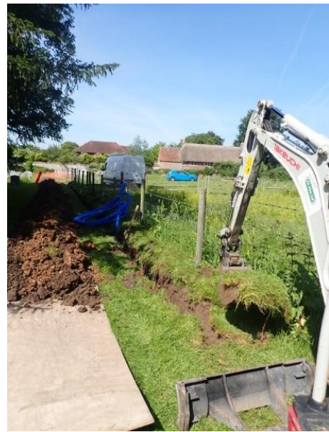
Plate 89: Excavation of the water pipe trench, from the east
