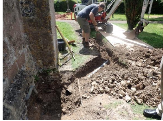
Plate 33: Excavation of the cable trench, from the north
