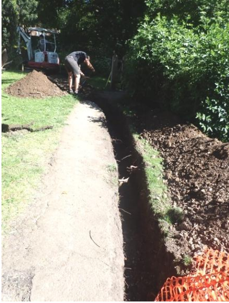
Plate 41: Excavation of the cable trench, from the south
