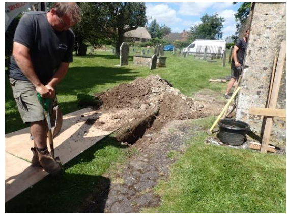
Plate 34: Excavation of the cable trench, from the south
