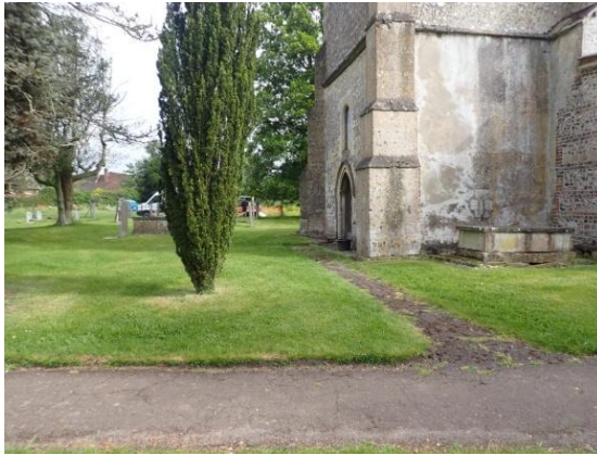
Plate 6: Pre-groundworks, from the south
