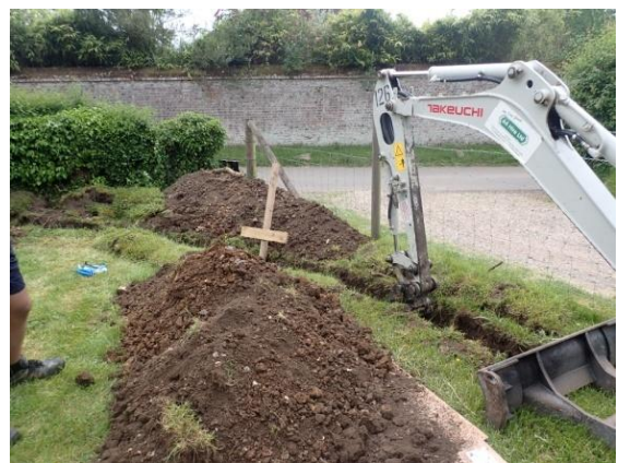
Plate 61: Excavation of the water pipe trench, from the east
