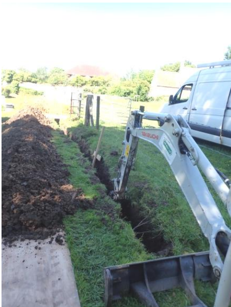
Plate 82: Excavation of the water pipe trench, from the east
