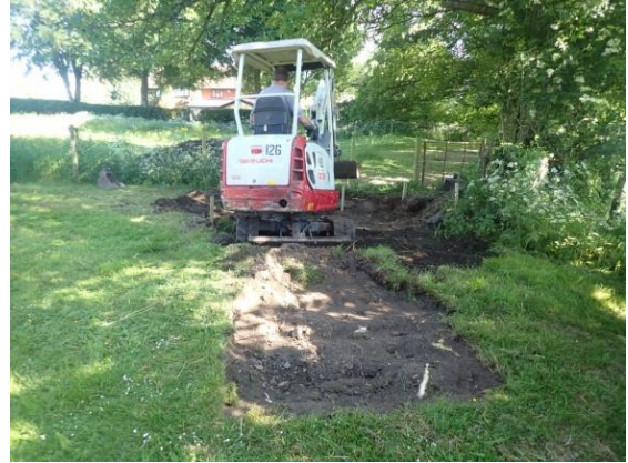
Plate 43: Excavation of the cable trench, from the south
