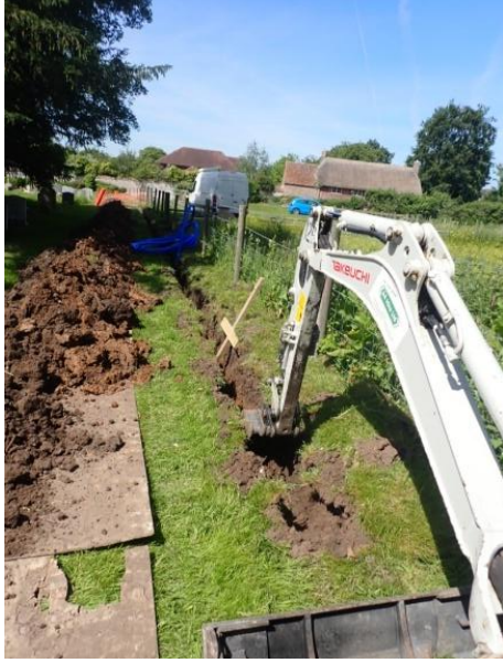
Plate 90: Excavation of the water pipe trench, from the east
