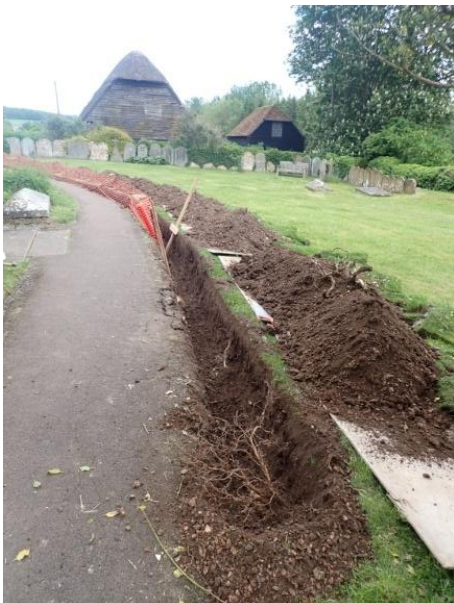
Plate 21: Excavation of the cable trench, from the west
