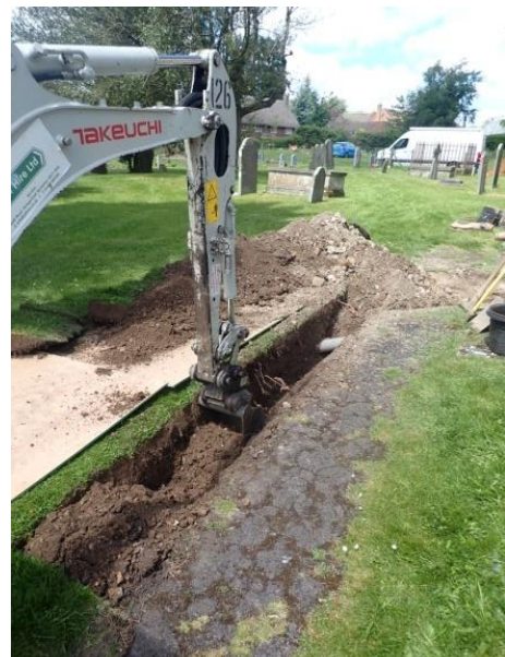
Plate 35: Excavation of the cable trench, from the south
