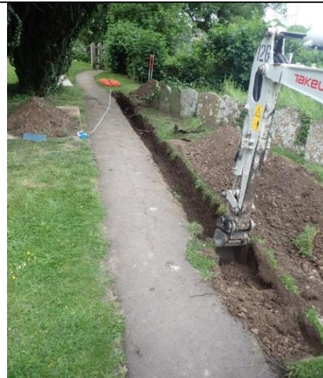
Plate 10: Excavation of the cable trench, from the south-west
