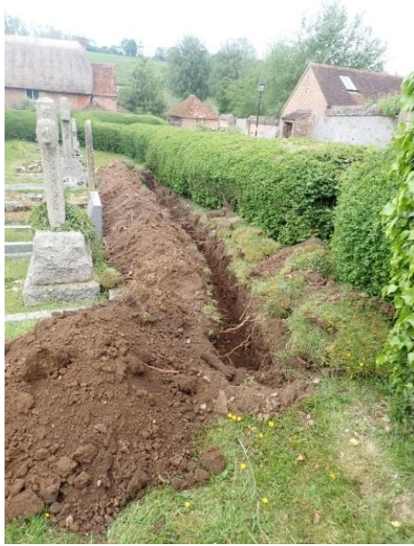
Plate 56: Excavation of the water pipe trench, from the north
