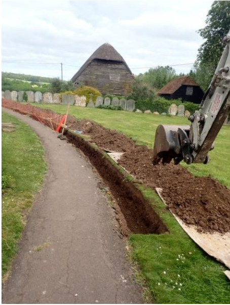
Plate 20: Excavation of the cable trench, from the west
