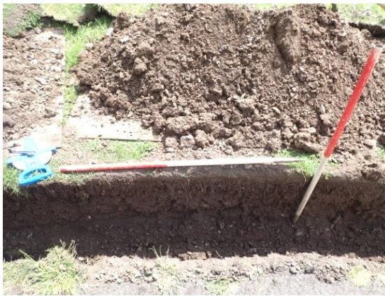
Plate 12: Representative Section 2, from the north-west
