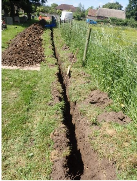
Plate 96: Excavation of the water pipe trench, from the east
