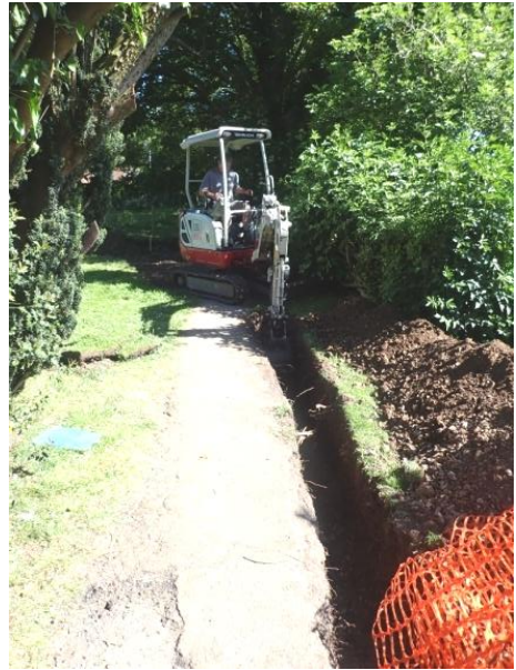
Plate 39: Excavation of the cable trench, from the south
