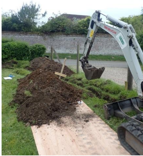
Plate 62: Excavation of the water pipe trench, from the east
