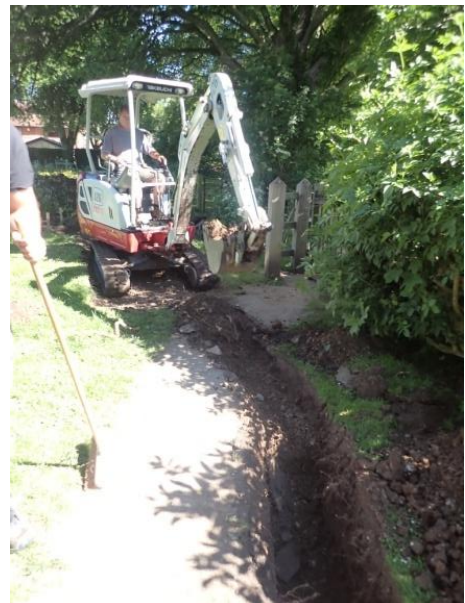
Plate 40: Excavation of the cable trench, from the south
