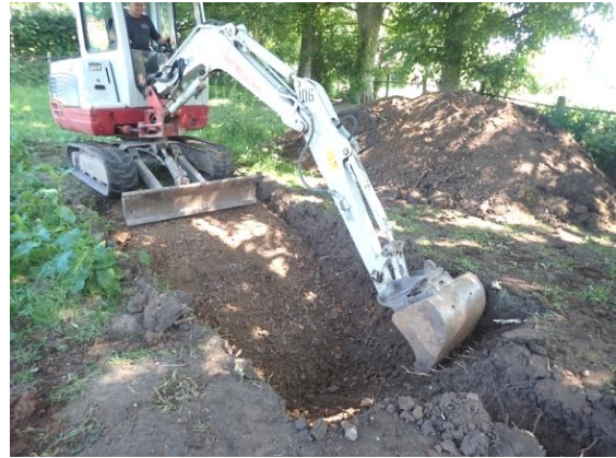
Plate 111: Excavations for the septic tank, from the south-west
