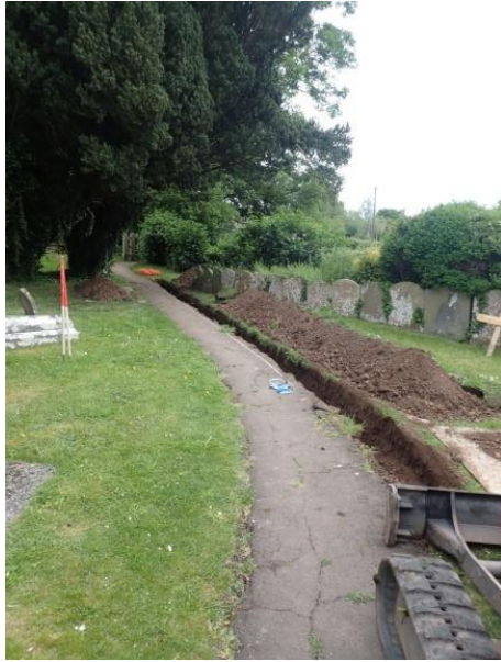
Plate 11: Excavation of the cable trench, from the south-west
