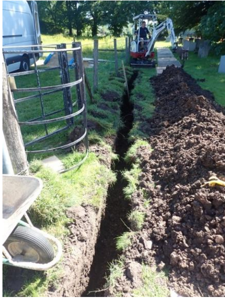
Plate 81: Excavation of the water pipe trench, from the west
