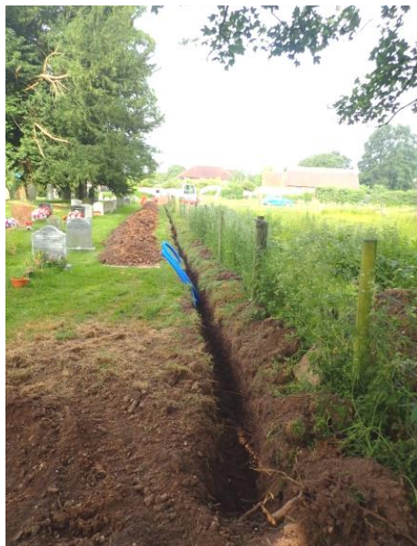
Plate 98: Excavation of the water pipe trench, from the east
