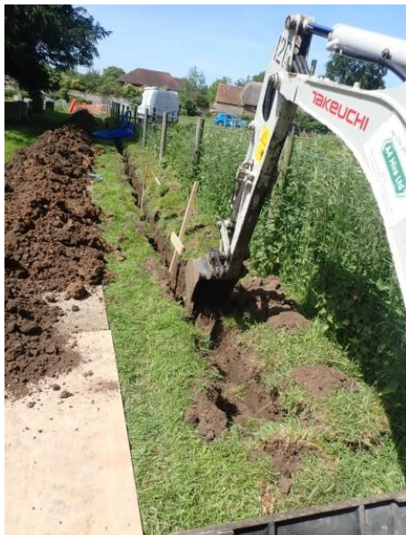
Plate 92: Excavation of the water pipe trench, from the east
