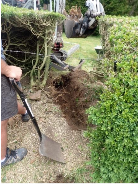
Plate 52: Excavation of the water pipe trench, from the west
