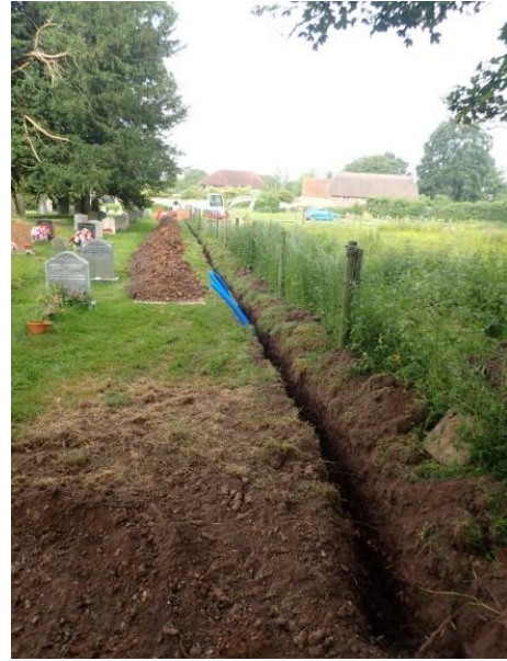
Plate 99: Excavation of the water pipe trench, from the east
