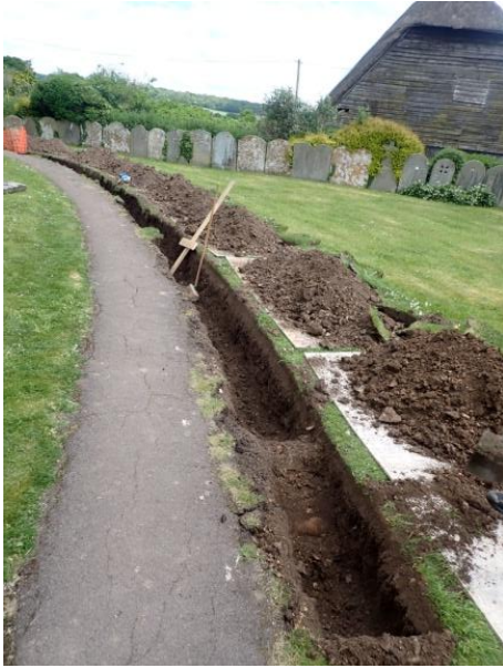
Plate 16: Excavation of the cable trench, from the west
