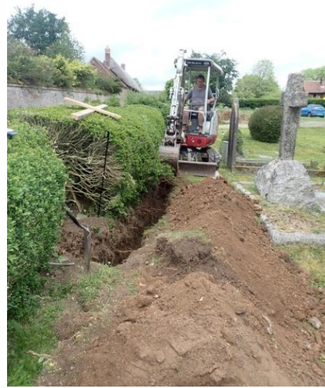
Plate 54: Excavation of the water pipe trench, from the south
