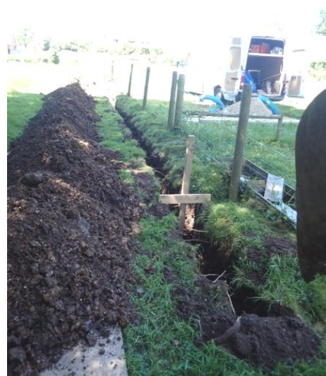
Plate 85: Excavation of the water pipe trench, from the east
