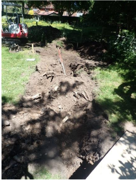
Plate 46: Excavation of the cable trench, from the south
