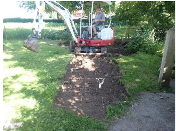
Plate 44: Excavation of the cable trench, from the south
