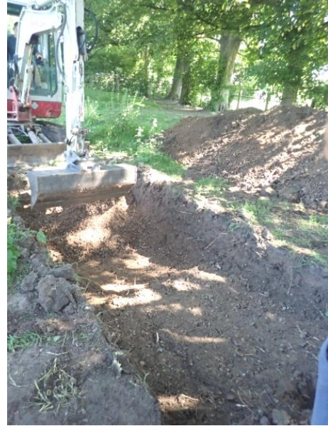
Plate 105: Excavations for the septic tank, from the south
