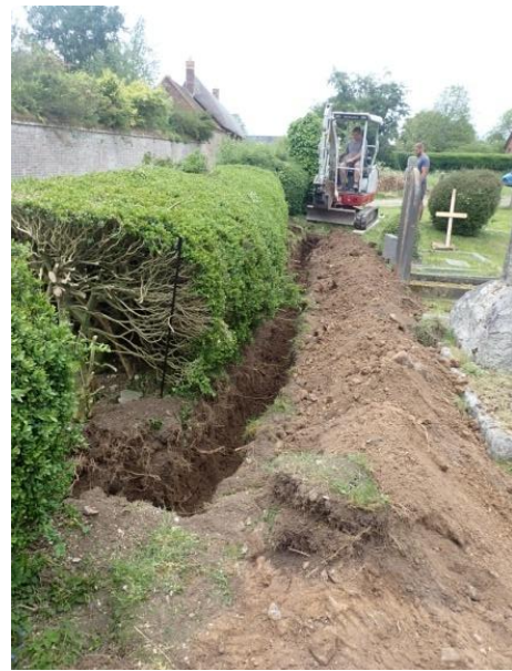
Plate 55: Excavation of the water pipe trench, from the south
