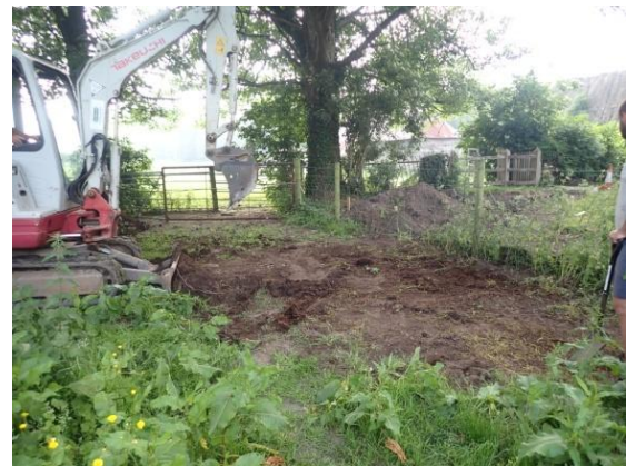
Plate 100: Excavations for the septic tank, from the south-west
