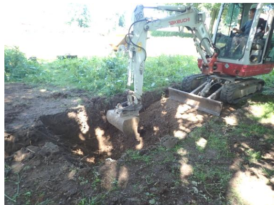
Plate 112: Excavations for the septic tank, from the east
