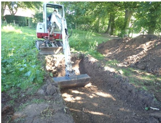
Plate 104: Excavations for the septic tank, from the south
