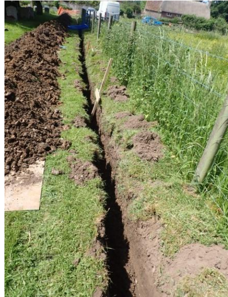
Plate 93: Excavation of the water pipe trench, from the east
