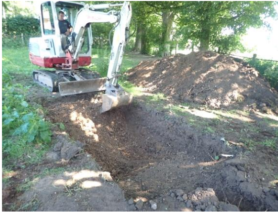
Plate 108: Excavations for the septic tank, from the south-west
