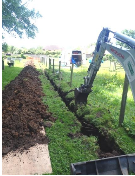
Plate 88: Excavation of the water pipe trench, from the east
