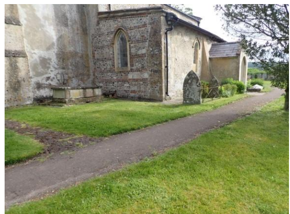
Plate 5: Pre-groundworks, from the south-west
