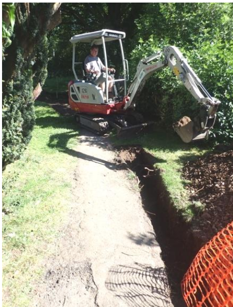
Plate 38: Excavation of the cable trench, from the south
