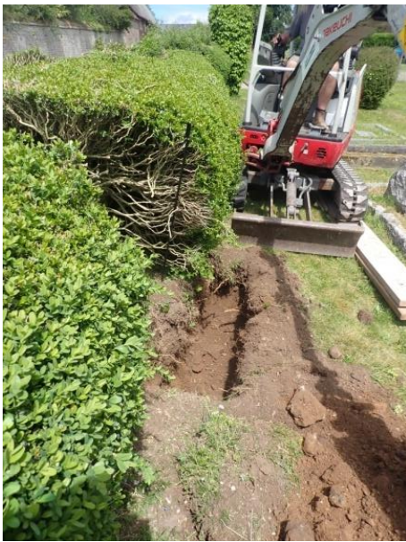
Plate 53: Excavation of the water pipe trench, from the south
