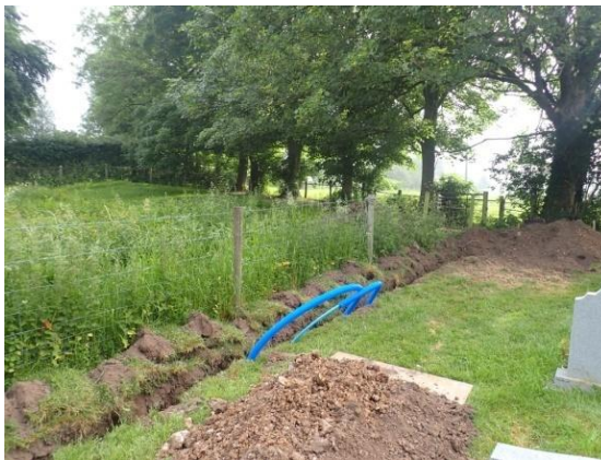
Plate 97: Excavation of the water pipe trench, from the south-west
