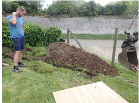
Plate 59: Excavation of the water pipe trench, from the south-east
