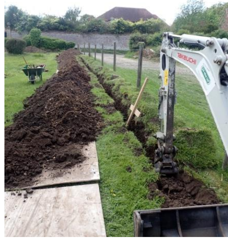
Plate 74: Excavation of the water pipe trench, from the east
