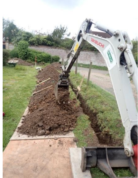
Plate 69: Excavation of the water pipe trench, from the east
