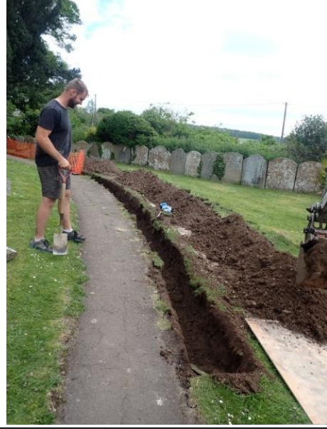
Plate 14: Excavation of the cable trench, from the west
