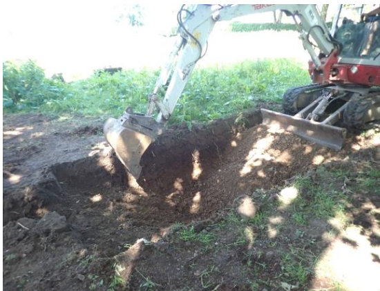
Plate 109: Excavations for the septic tank, from the east
