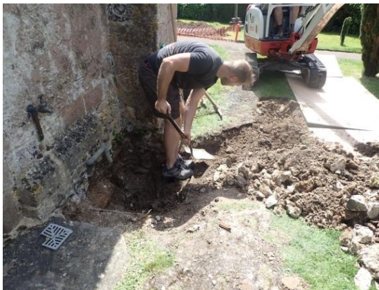
Plate 32: Excavation of the cable trench, from the north
