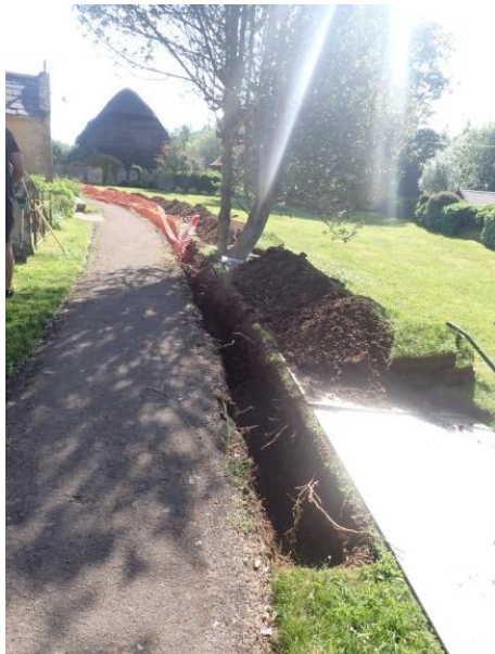
Plate 26: Excavation of the cable trench, from the west
