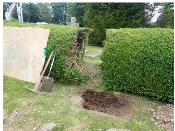
Plate 51: Excavation of the water pipe trench, from the west
