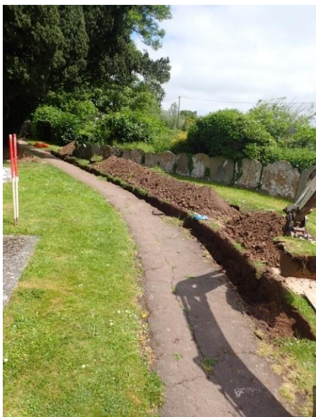
Plate 13: Excavation of the cable trench, from the south-west
