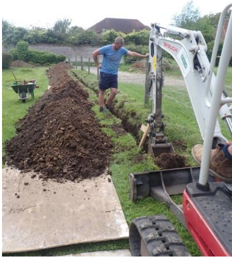
Plate 72: Excavation of the water pipe trench, from the east
