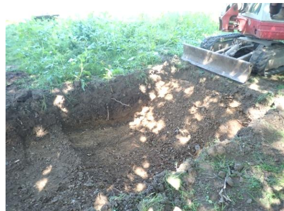
Plate 107: Excavations for the septic tank, from the east
