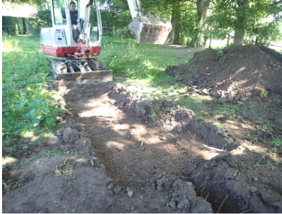
Plate 102: Excavations for the septic tank, from the south
