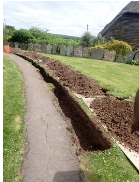
Plate 15: Excavation of the cable trench, from the west
