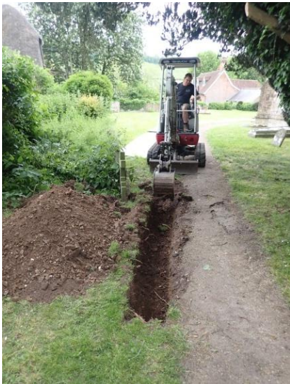
Plate 7: Excavation of the cable trench, from the north
