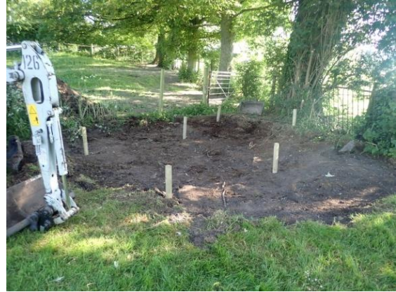
Plate 49: Excavated toilet block site, from the south
