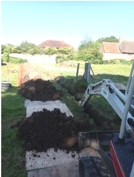
Plate 77: Excavation of the water pipe trench, from the east
