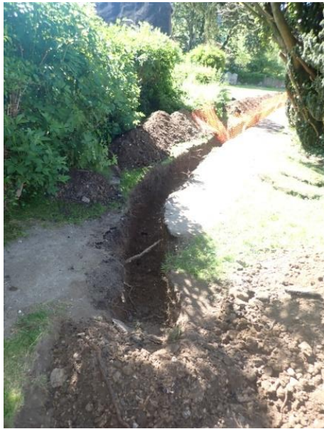
Plate 42: Excavation of the cable trench, from the south
