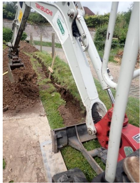
Plate 65: Excavation of the water pipe trench, from the east
