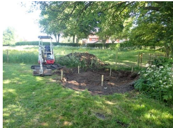
Plate 50: Excavated toilet block site, from the south-east
