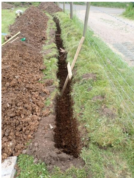
Plate 67: Excavation of the water pipe trench, from the east
