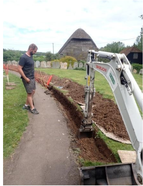
Plate 18: Excavation of the cable trench, from the west
