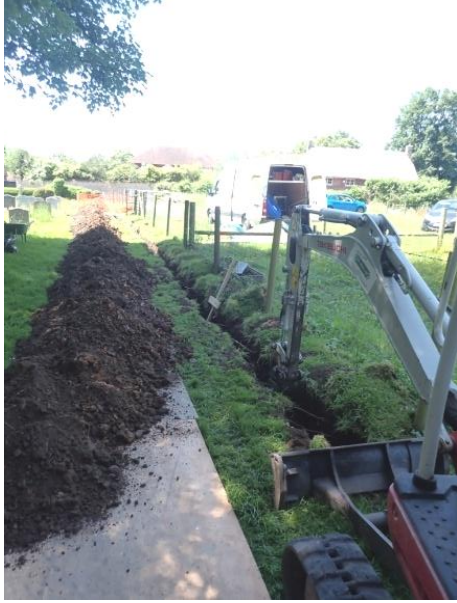
Plate 86: Excavation of the water pipe trench, from the east
