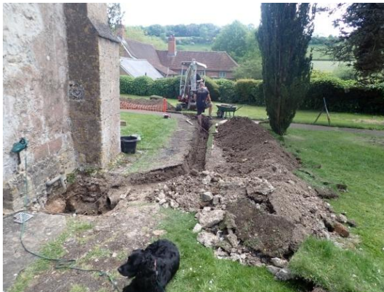
Plate 37: Excavation of the cable trench, from the north
