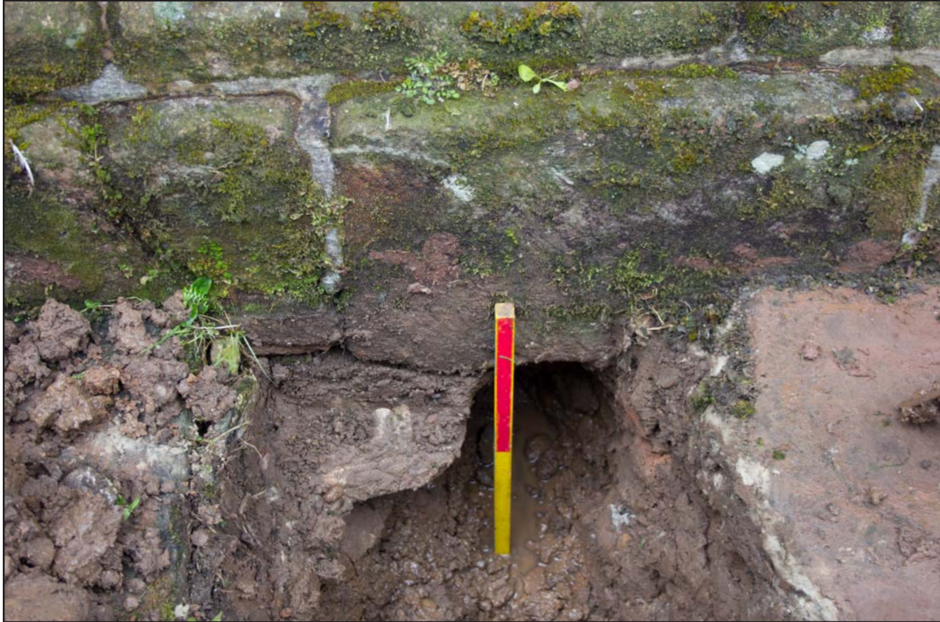
Plate 10: Test pit 4 showing church wall foundations, from the north. Scale 0.5m.
