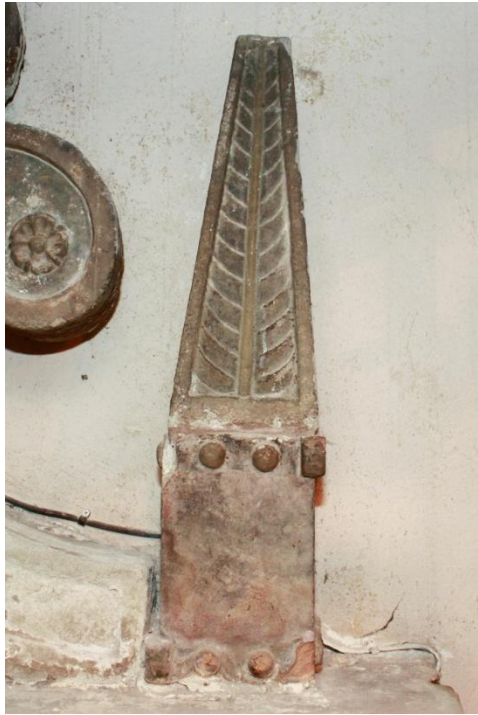
The viewer's right-hand pinnacle at entablature level, before and after cleaning. Note the delicately applied, green decoration is not apparent before conservation and will be difficult to establish from floor-level, with the current ambient lighting. Note also the black horizontal banding complete with gilded spherical domes above and below the red marbling, complete with black veining.
