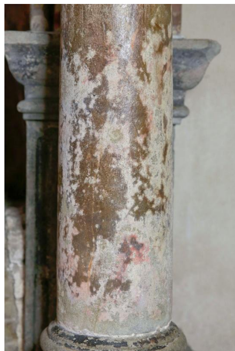
The extent of deterioration to the bottom of the right-hand column. Loss has been caused by physical wear being at low-level, likely - intentional over-cleaning, and the effects of efflorescence. Note how the cleaning process has imparted a degree of lustre, back to the degraded, aged paint.
