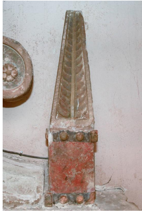
The viewer's right-hand pinnacle at entablature level, before and after cleaning. Note the delicately applied, green decoration is not apparent before conservation and will be difficult to establish from floor-level, with the current ambient lighting. Note also the black horizontal banding complete with gilded spherical domes above and below the red marbling, complete with black veining.
