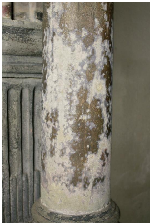
The extent of deterioration to the bottom of the right-hand column. Loss has been caused by physical wear being at low-level, likely - intentional over-cleaning, and the effects of efflorescence. Note how the cleaning process has imparted a degree of lustre, back to the degraded, aged paint.
