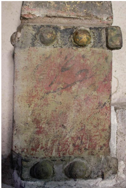
The marbling with black veining (as in real marble) is more apparent after cleaning, as is the oil-gilding, which highlights the extent of care and cost lavished on an otherwise more humble sandstone monument.
