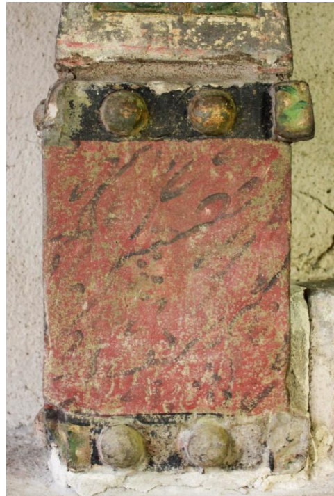
The marbling with black veining (as in real marble) is more apparent after cleaning, as is the oil-gilding, which highlights the extent of care and cost lavished on an otherwise more humble sandstone monument.
