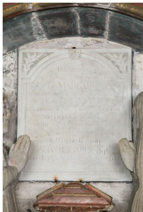
The later, lightly-incised, marble dedication panel in the recess, during and after cleaning. The marble responded well to a solvent mixture. It could have been taken much further and re-polished, but that approach is inappropriate, choosing instead a light-general clean. Note the top of the lectern between the two kneeling figures is completely cleaned in this image, revealing the crude marbling to the painted, carved sandstone.
