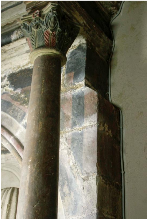
The right-hand column and spandrel (behind) before and after cleaning. Note the thick, vertical black-line looks like a shadow, but has been painted intentionally. The marbling to the column would have looked realistic when first applied (before deterioration) and only looks obvious now, due to the loss of paint at the bottom, exposing the sandstone beneath.
