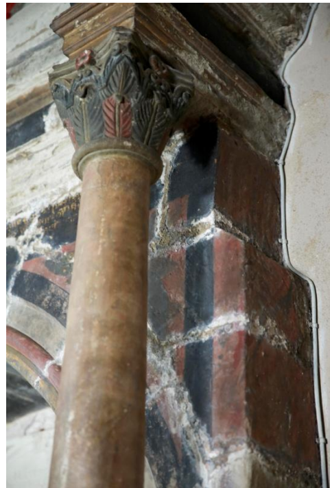
The right-hand column and spandrel (behind) before and after cleaning. Note the thick, vertical black-line looks like a shadow, but has been painted intentionally. The marbling to the column would have looked realistic when first applied (before deterioration) and only looks obvious now, due to the loss of paint at the bottom, exposing the sandstone beneath.
