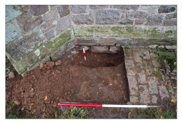
Photo 3. General view of Trial Pit 1, looking S. The compacted pebble fill (4) has been excavated, exposing the foundation trench cut [5].
