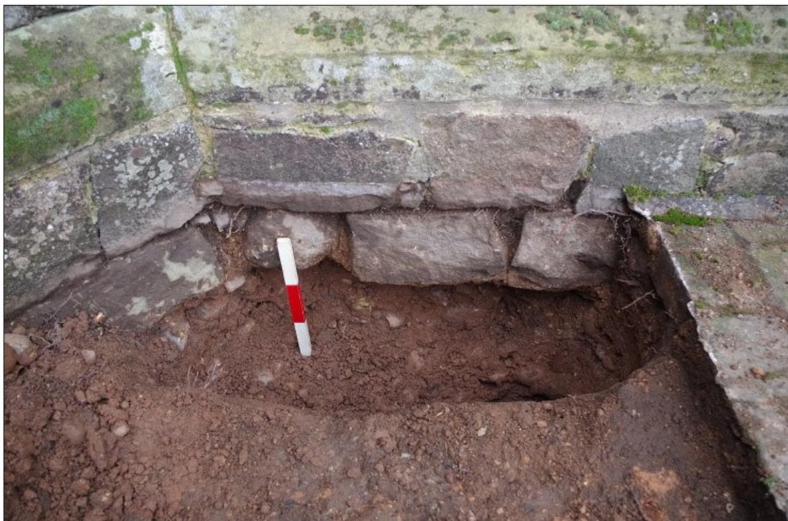
Photo 4. Trial Pit 1, showing lower course of north chancel wall above fill (4) of foundation trench [5], looking S.
