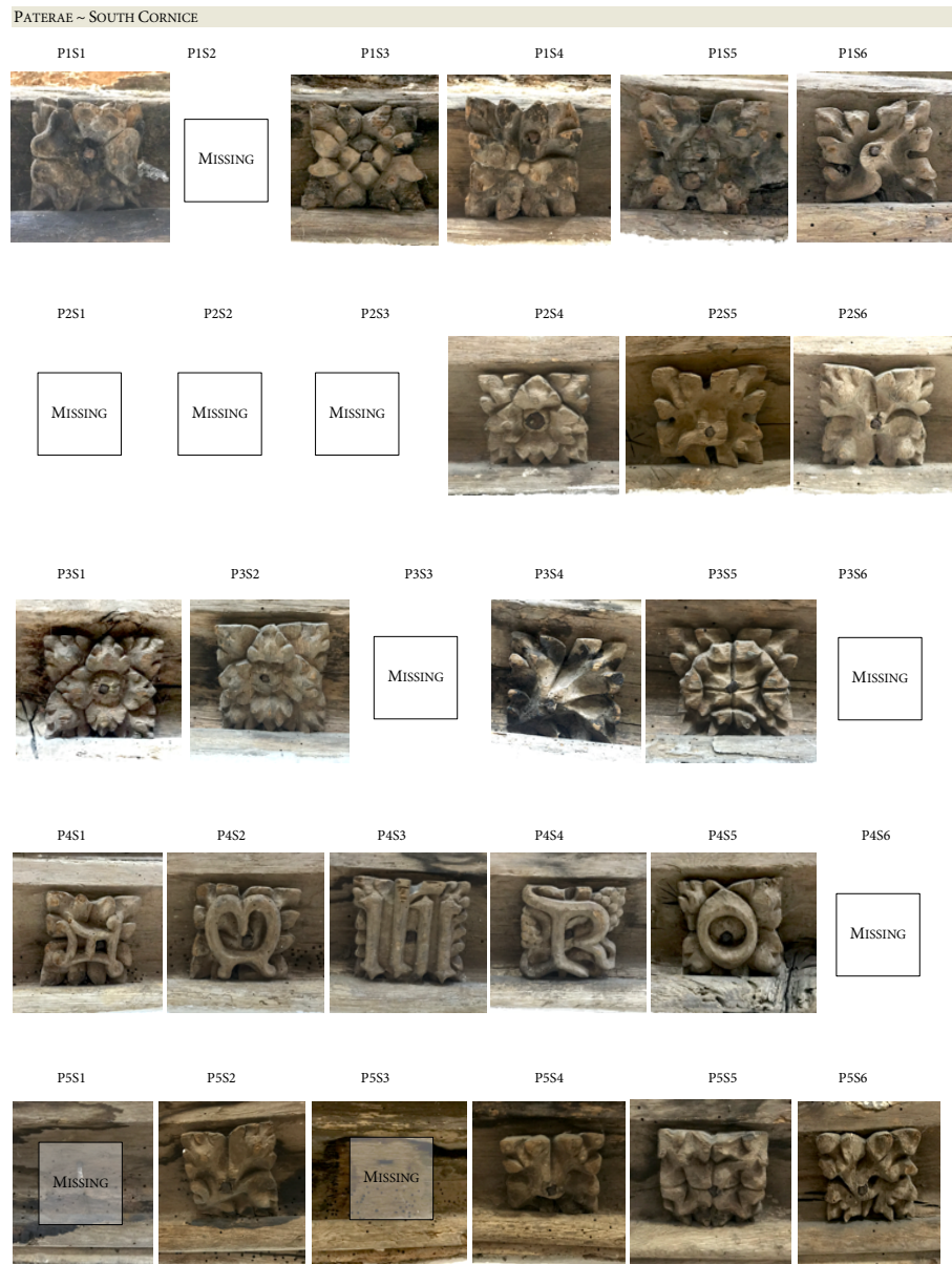
Figure 6 ~ Paterae on the south elevation timber cornice.
