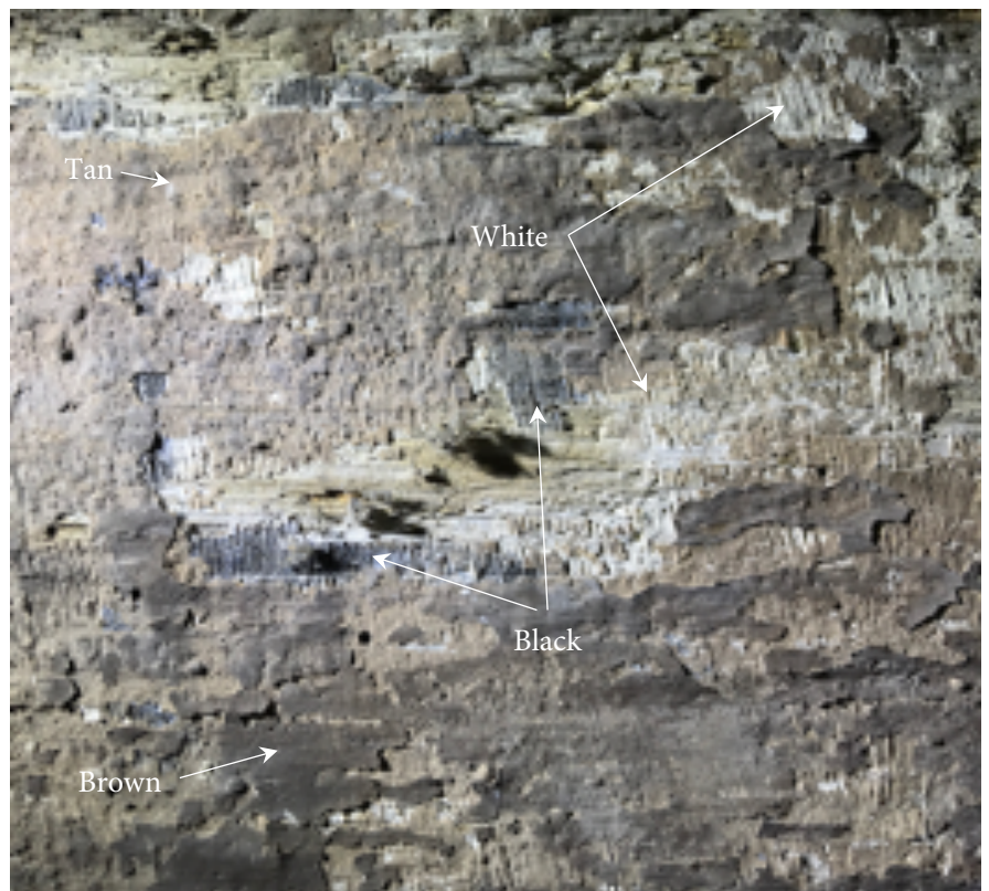
Figure 10 ~ Detail of painted area on Truss 9 in raking light illustrating the vertical brush strokes of the underlying white and black paint applications.
