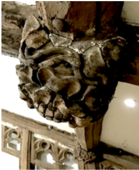
Figure 21 ~ Repair of the wallplate of Bay 5 South elevation.
