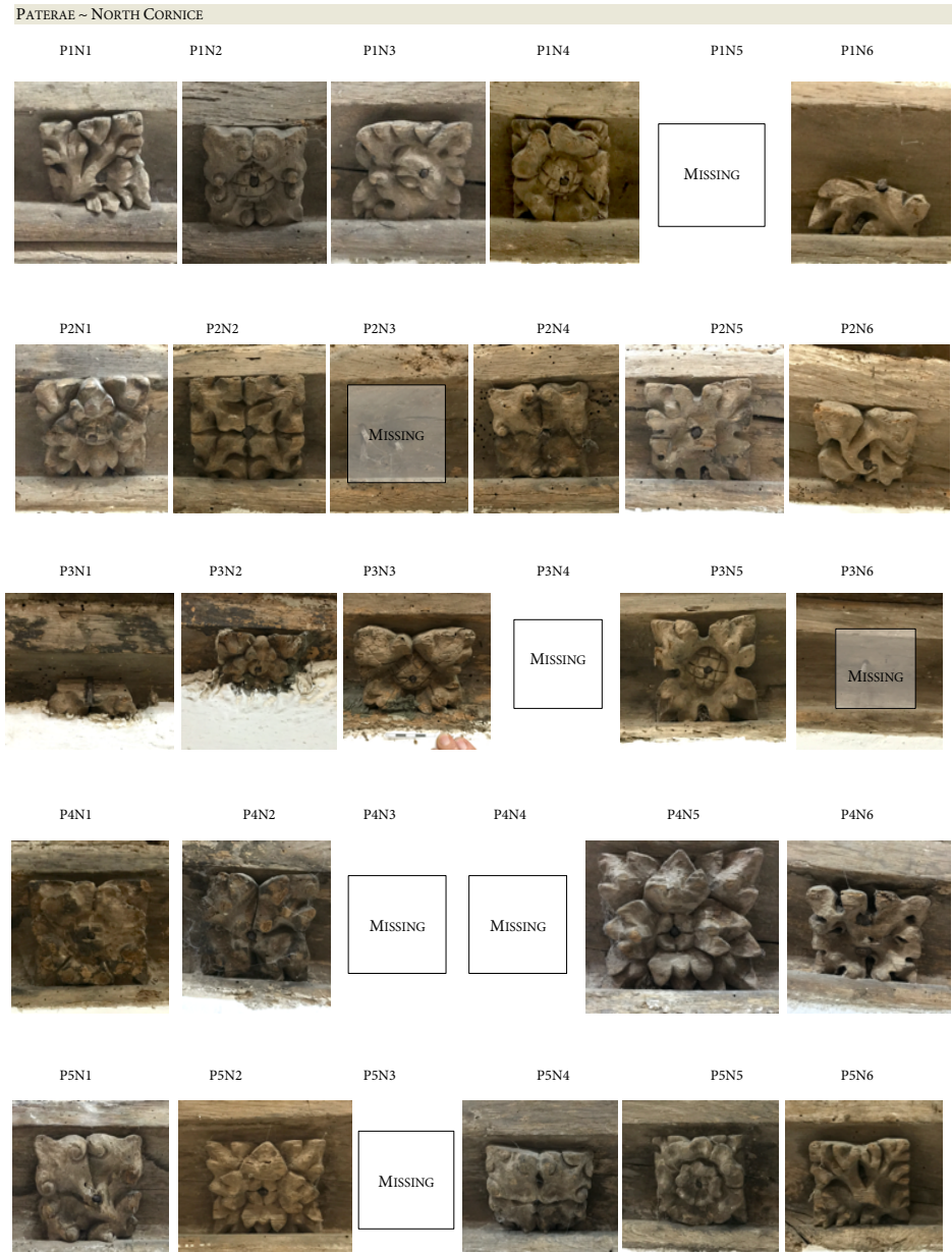
Figure 5 ~ Paterae on the north elevation timber cornice.
