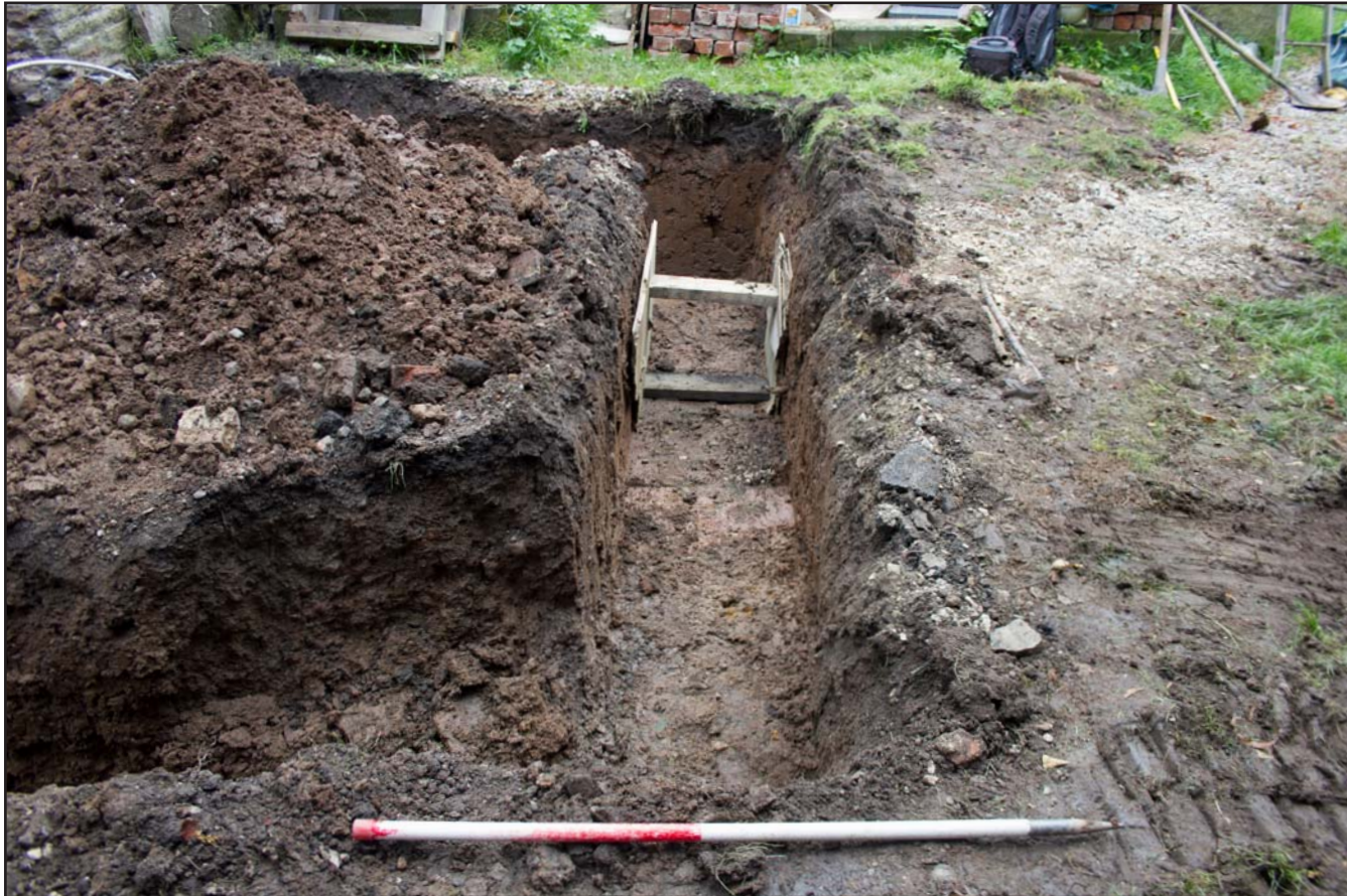
Plate 05: Trench 2 post excavation at St. Mary's Church, Bosley, Macclesfield - from the west - scale 1m
