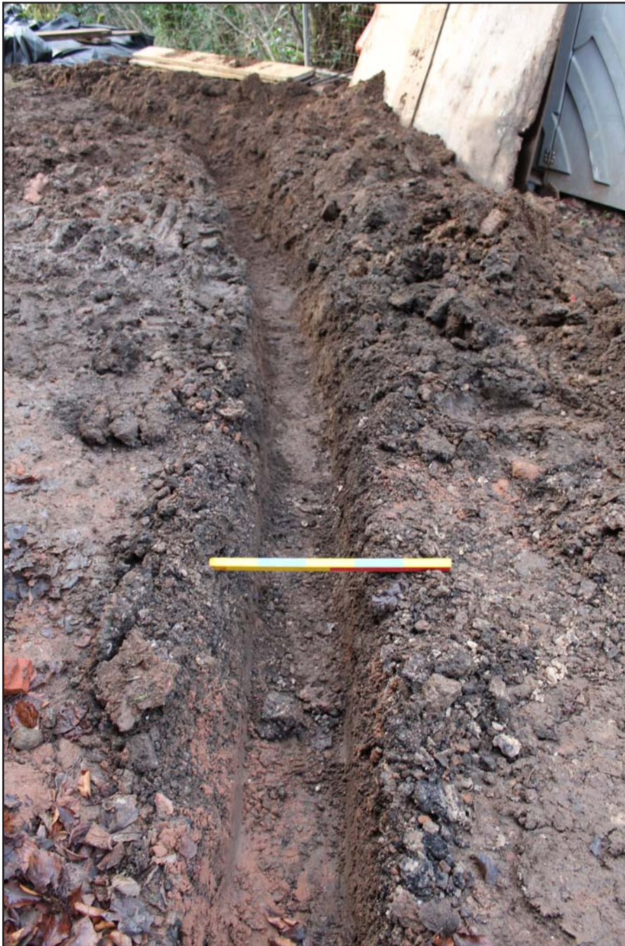
Plate 21: Large drain post excavation at St. Mary's Church, Bosley, Macclesfield - from the north - 0.50m scale
