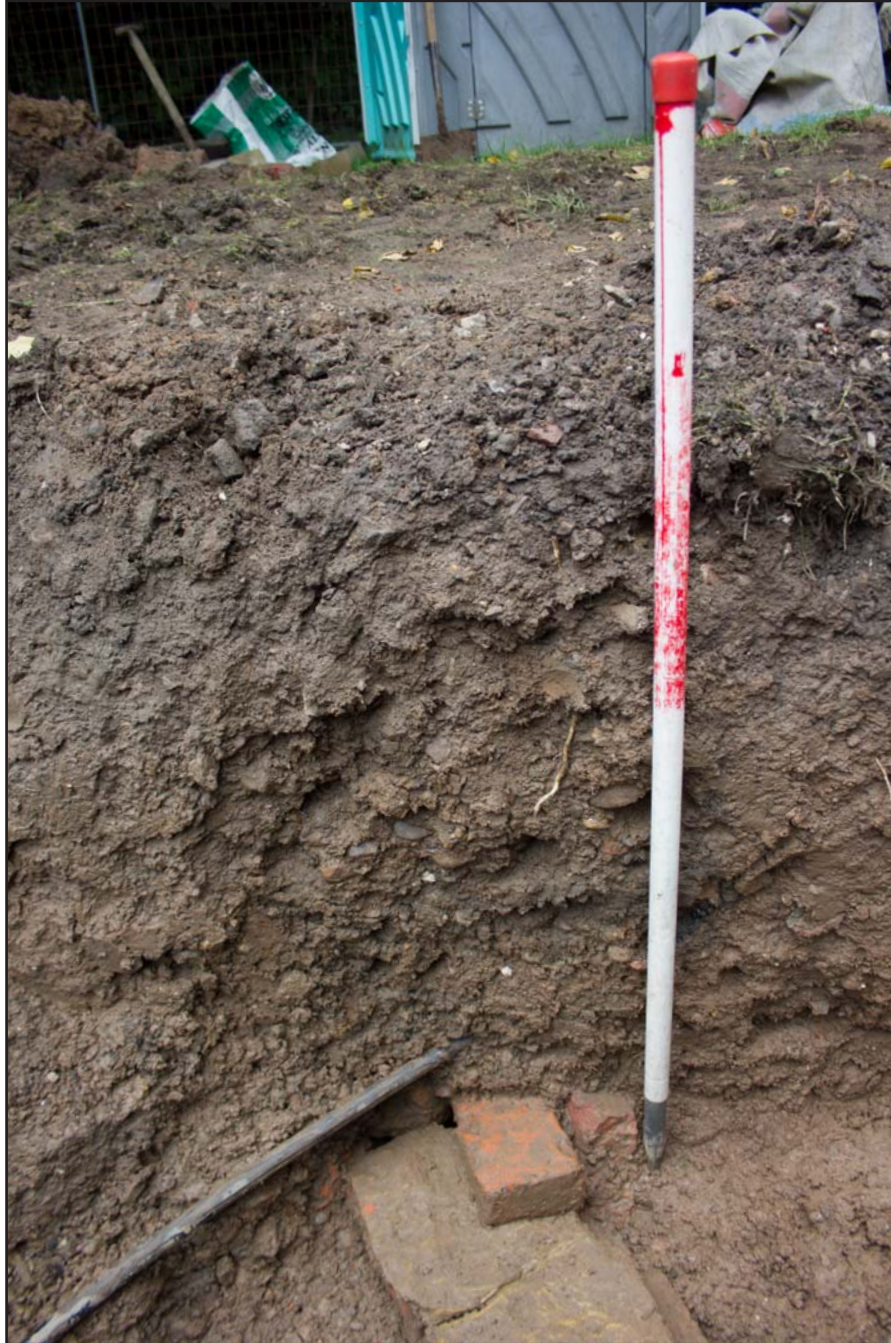
Plate 08: Section of Trench 3 showing placement of stone-capped brick culvert at St. Mary's Church, Bosley, Macclesfield - from the east - scale 1m
