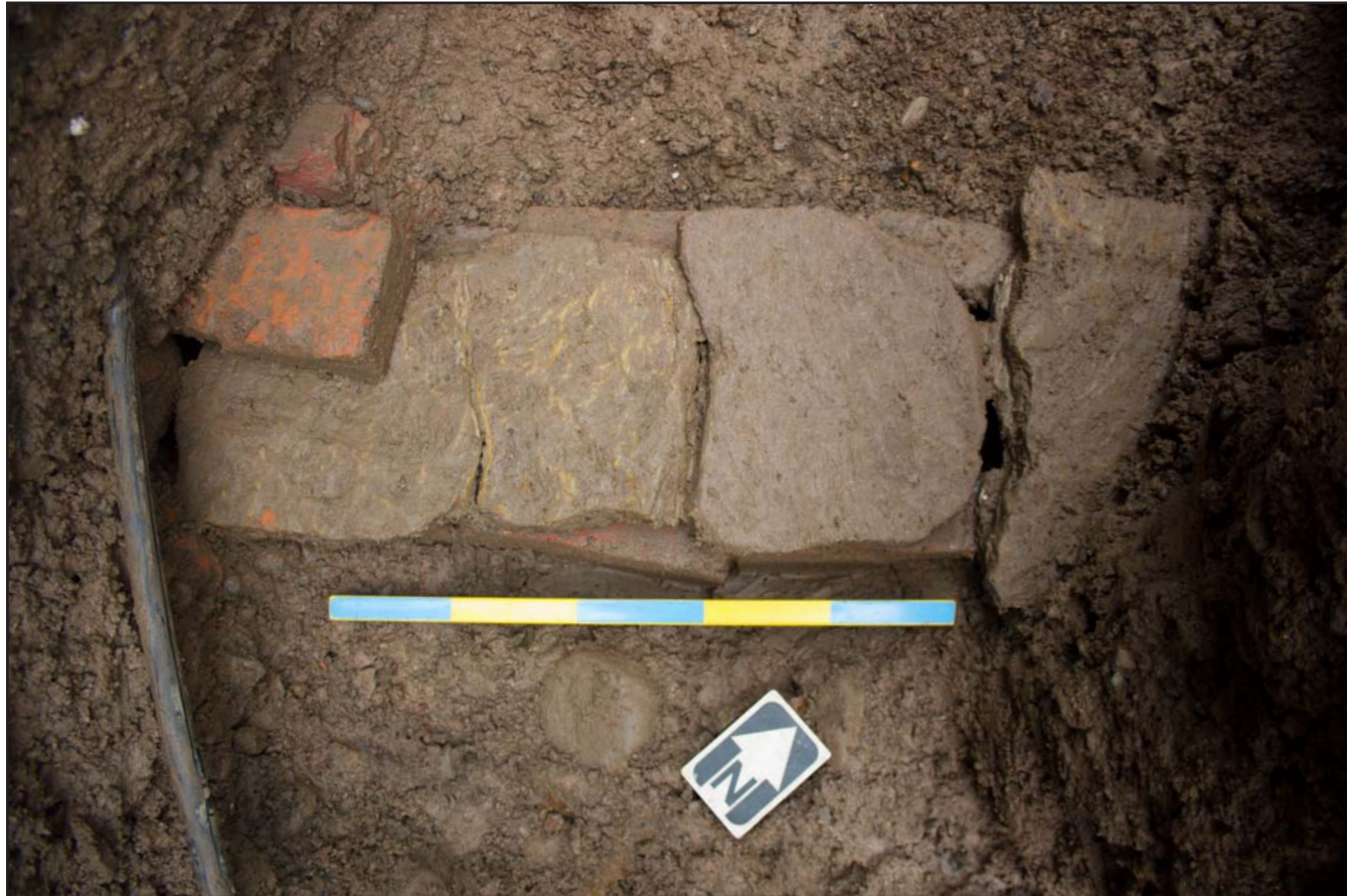
Plate 09: Stone-capped brick culvert in plan at St. Mary's Church, Bosley, Macclesfield - from the southeast - scale 0.50m
