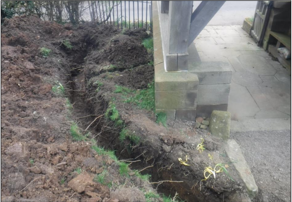
Plate 1. Eastern part of trench within graveyard, looking east.
