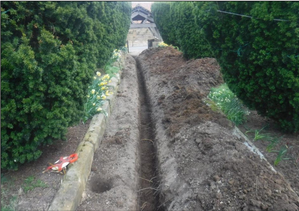
Plate 3. Trench within gravel path, looking east.
